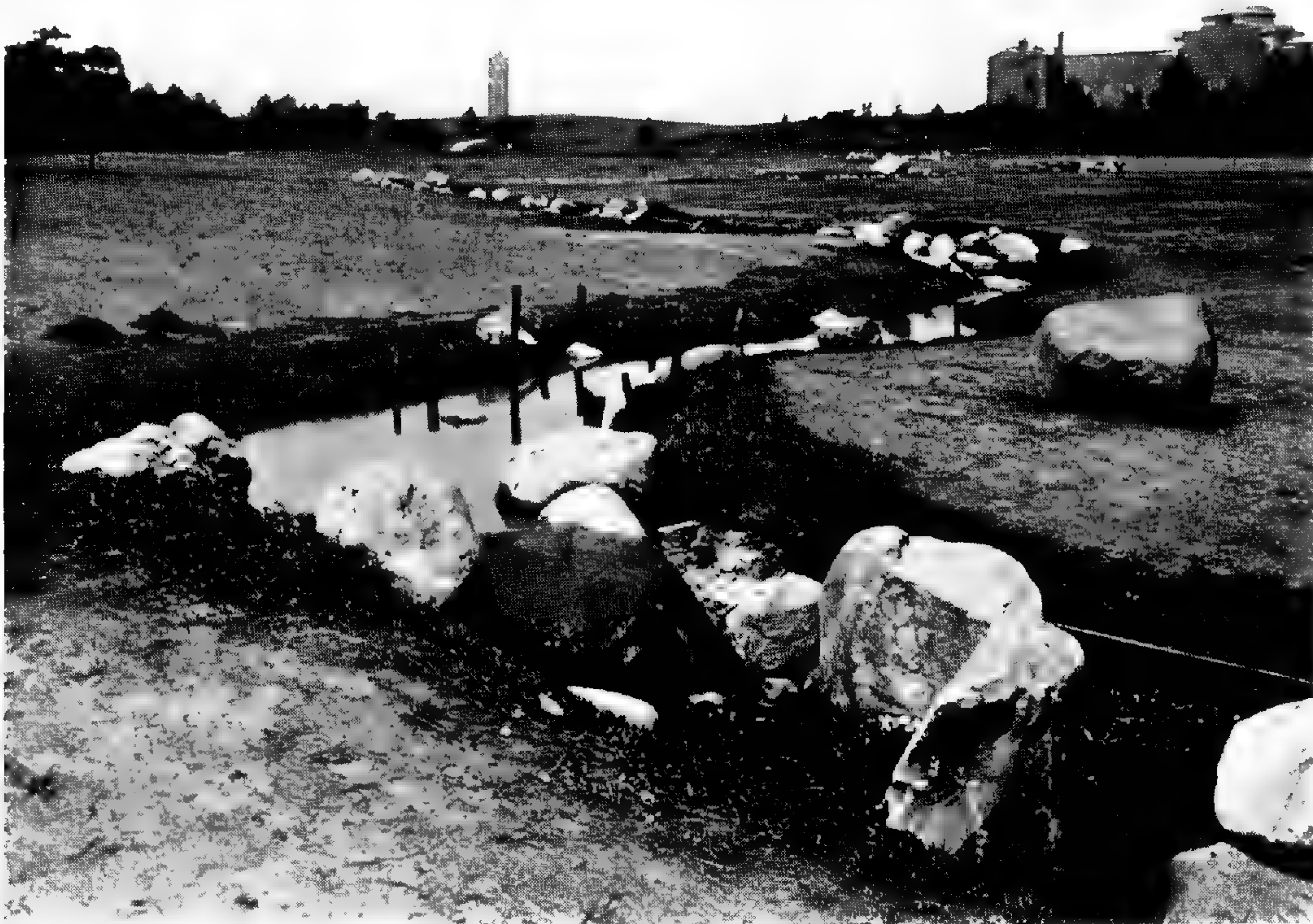
FIG. 4. Glacial boulders placed along the Brook under construction, 1912. Facing north—up stream. (562). Cf. Fig. 1.
