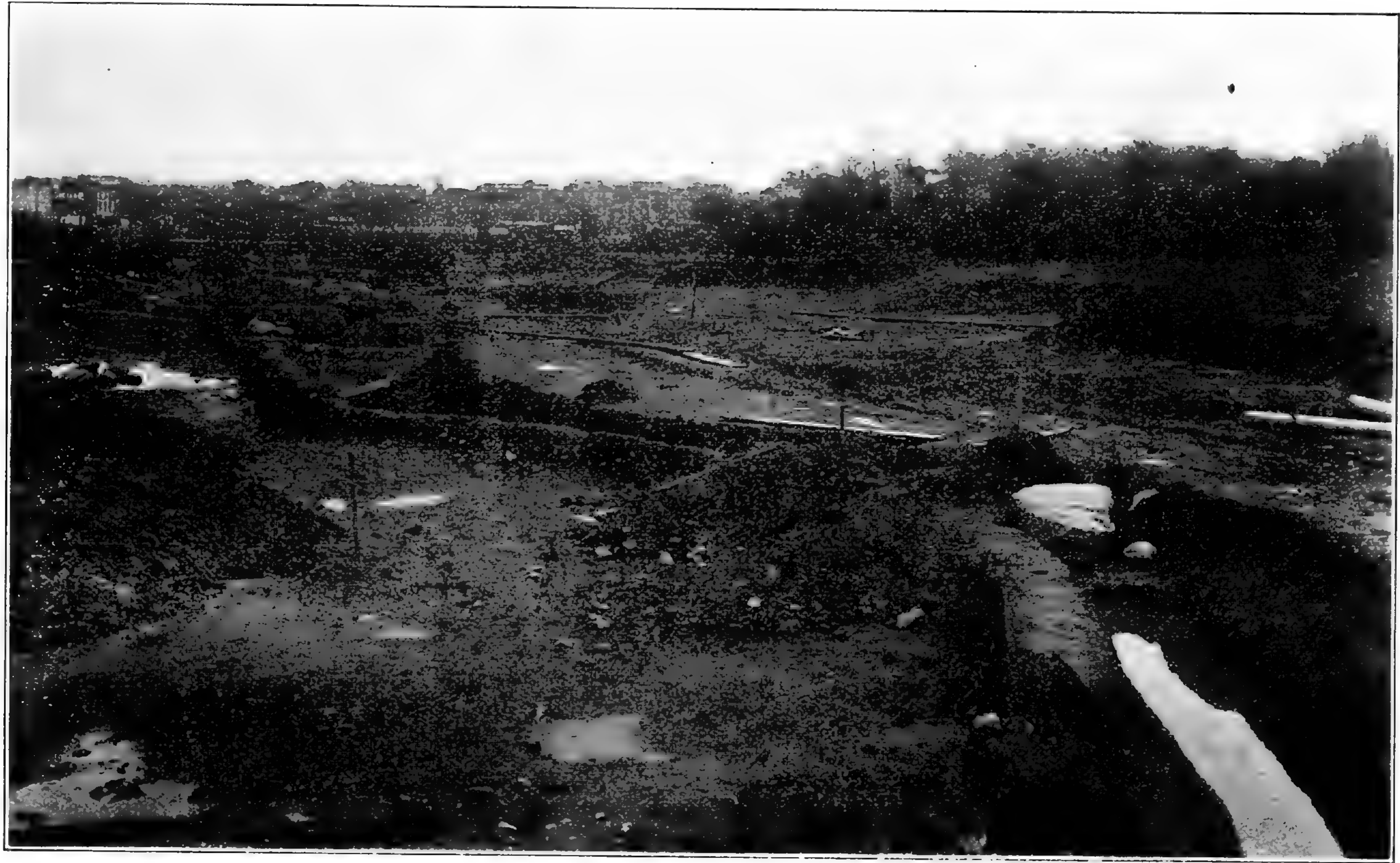
FIG. 14. View looking south along the brook, May 9, 1912, showing depth of excavation, and the locus of the swamp at the left middle distance. The mounds of soil around the surveyor's stakes show the level of the surface before grading.
