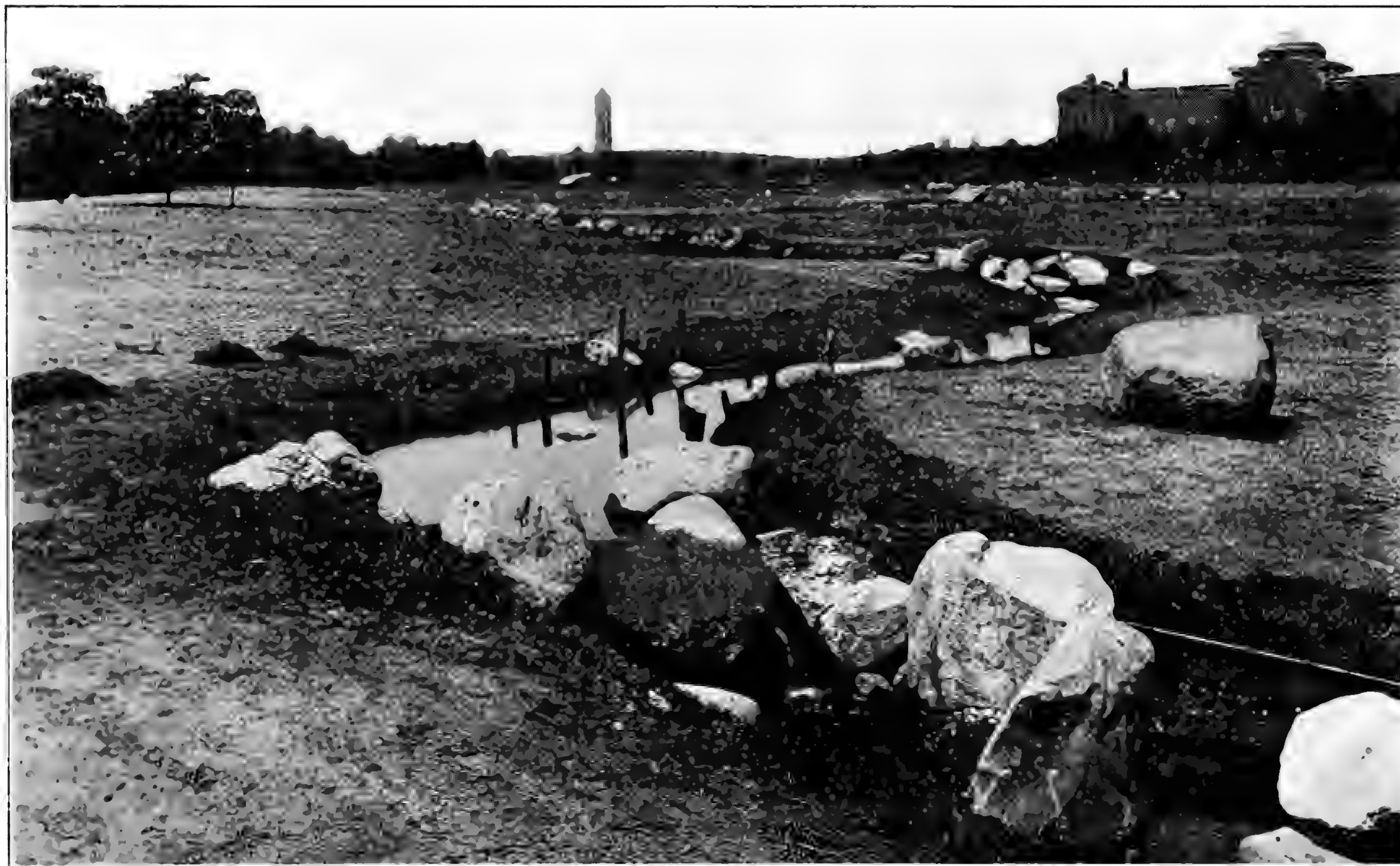
FIG. 13. View along the brook, July 25, 1912, looking north from just below dam No. 5. All boulders shown were transported from elsewhere by the laborers.
