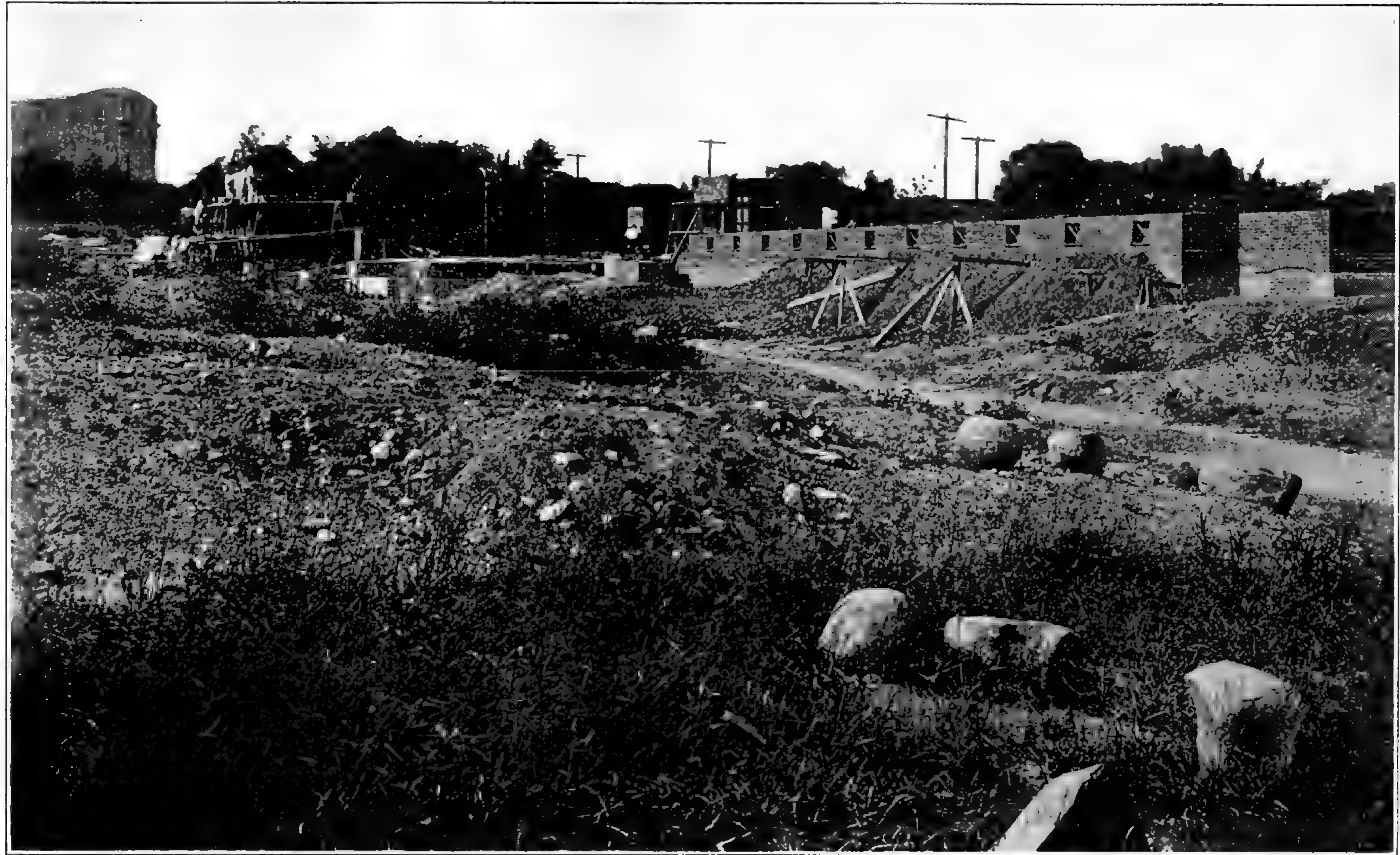
FIG. 7. Beginning the superstructure. Laboratory building and conservatories; Section 1. July 22, 1912.
