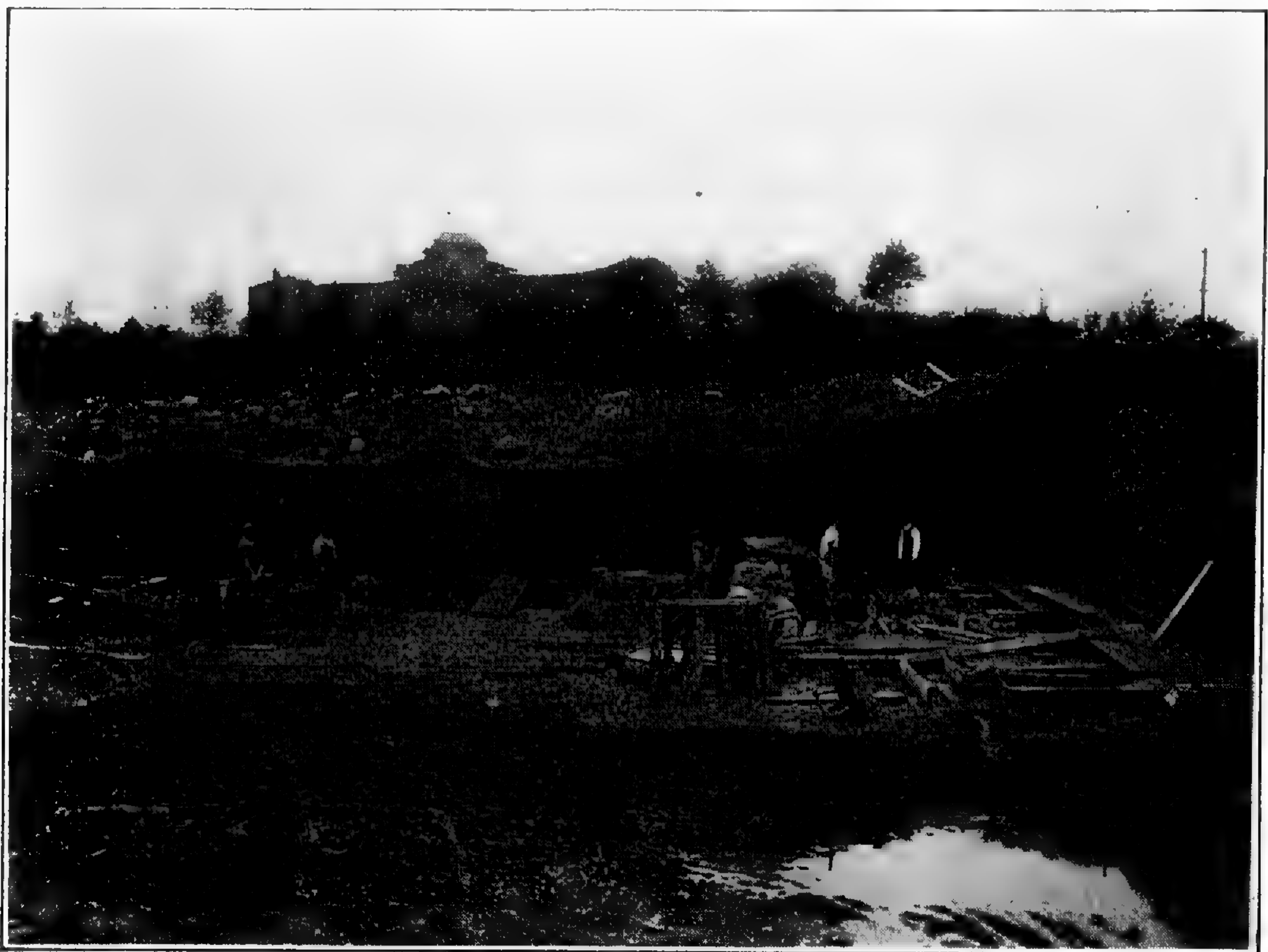
FIG. 6. Laying the foundations for Section I of the laboratory building. May 9, 1912.
