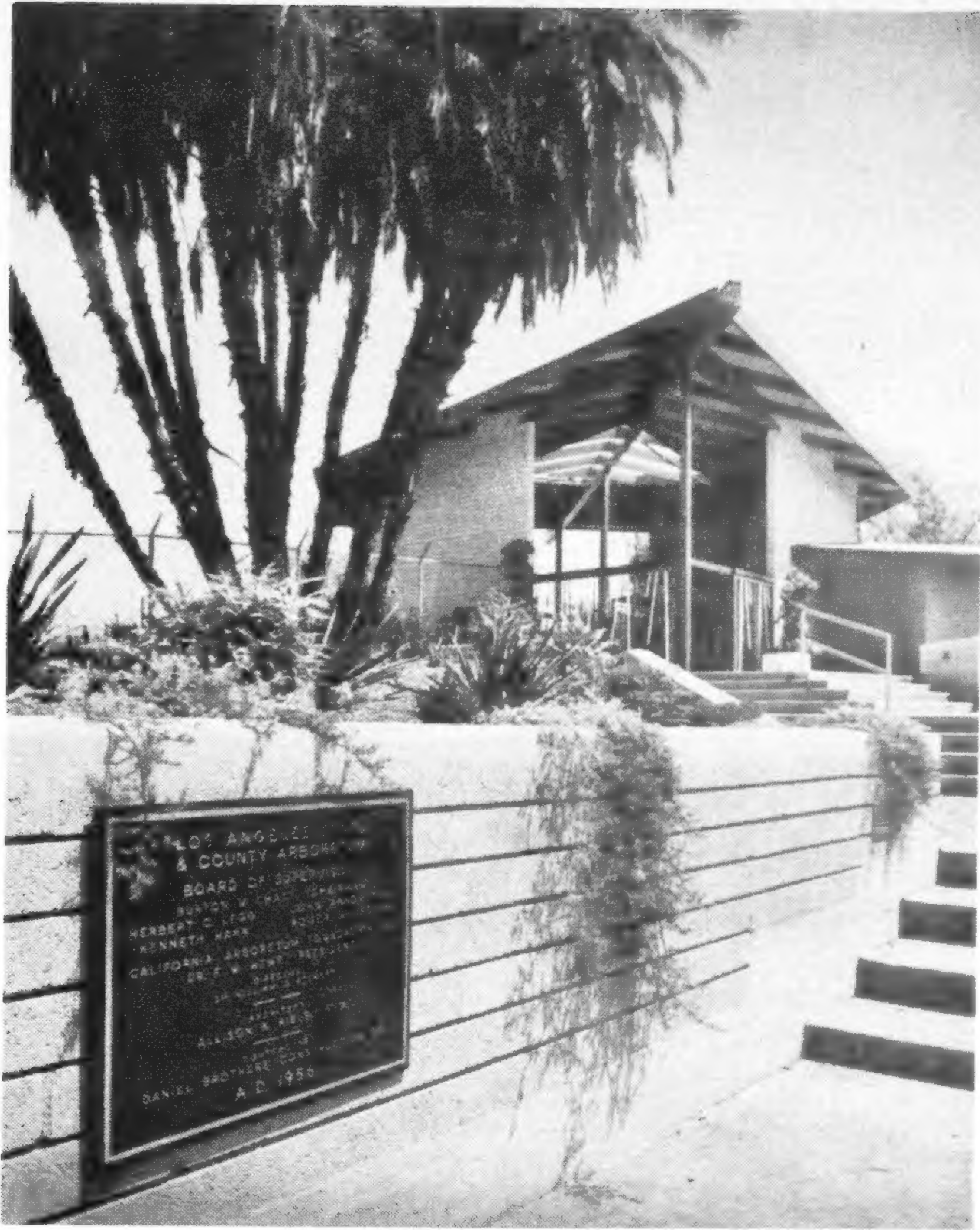
Stairway and entrance to the Administration Building.
