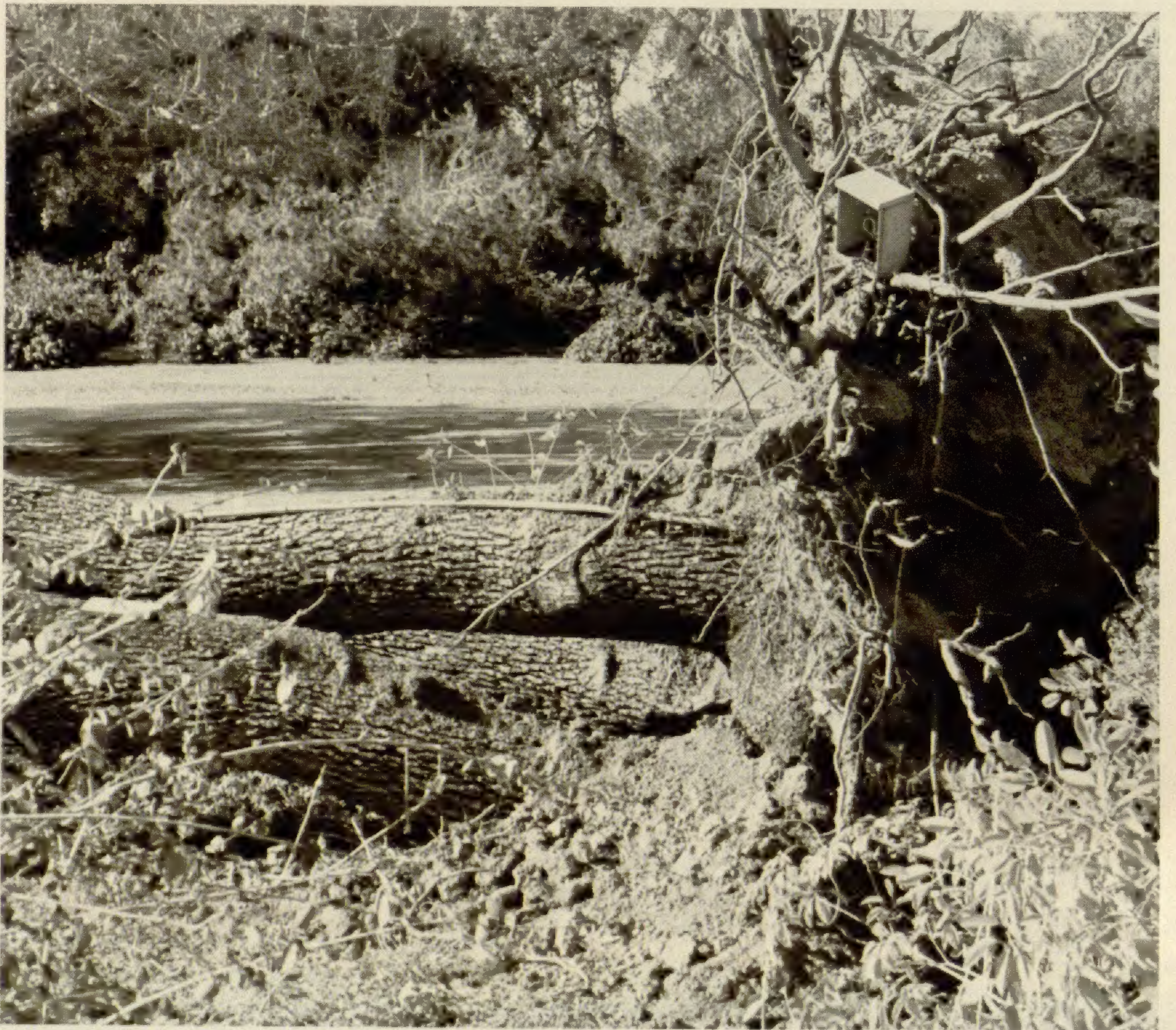
Electrical circuits on Tallac Knoll were disrupted when the old oak tree supporting the wiring blew over.
