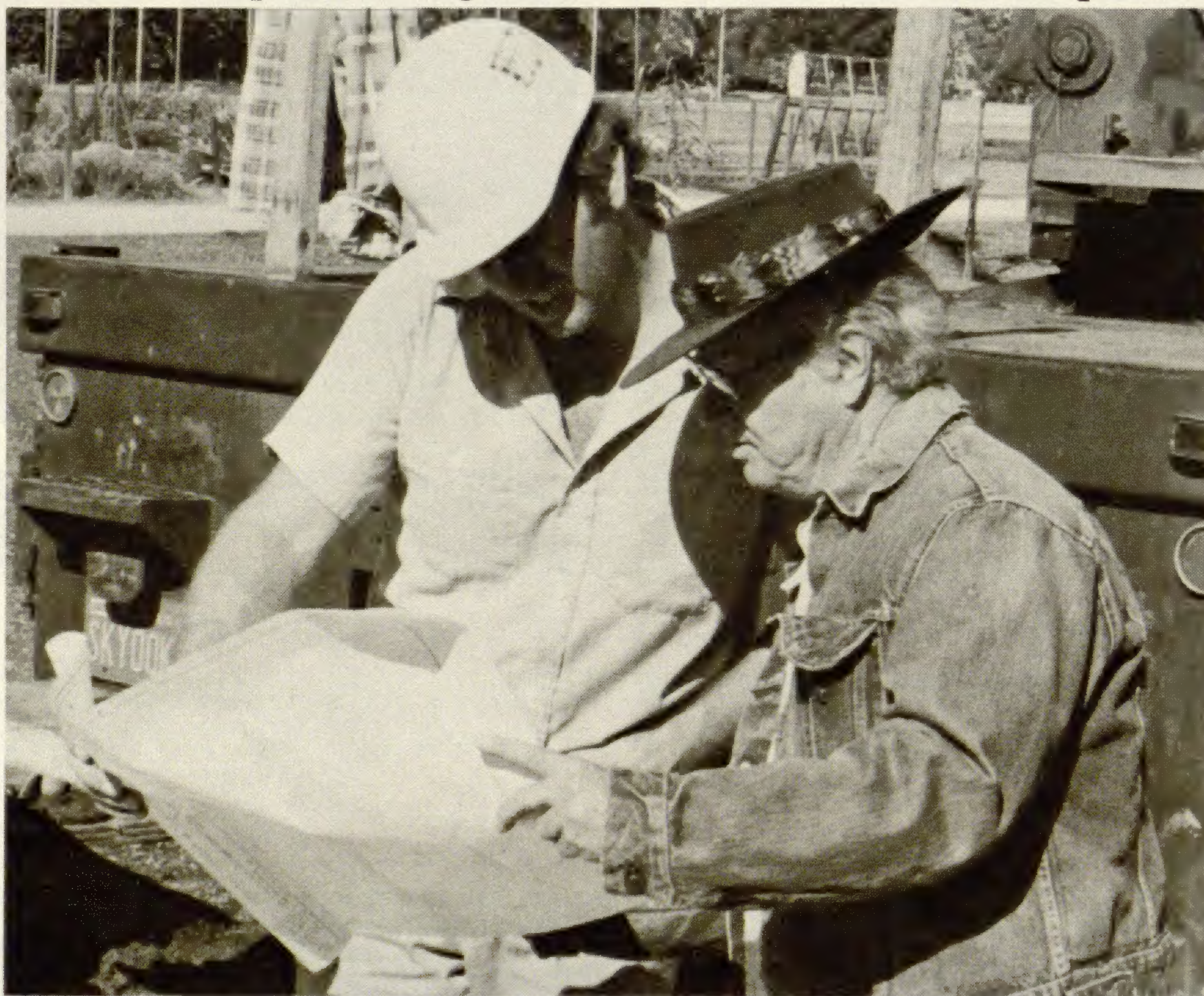
Mark Galbraith (left) and his father, John, check plans as a crane begins lifting the ramada beams into place.
