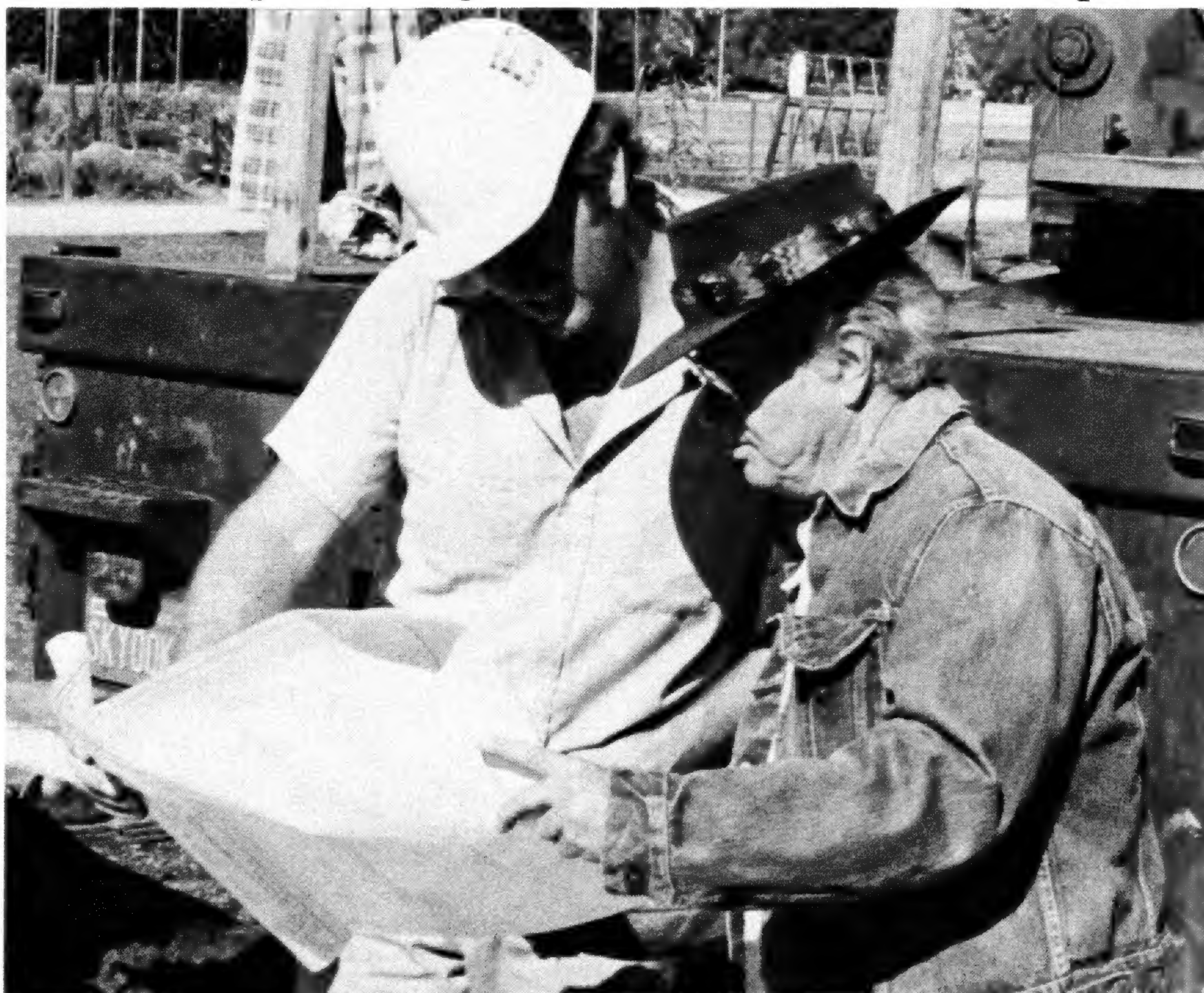
Mark Galbraith (left) and his father, John, check plans as a crane begins lifting the ramada beams into place.
