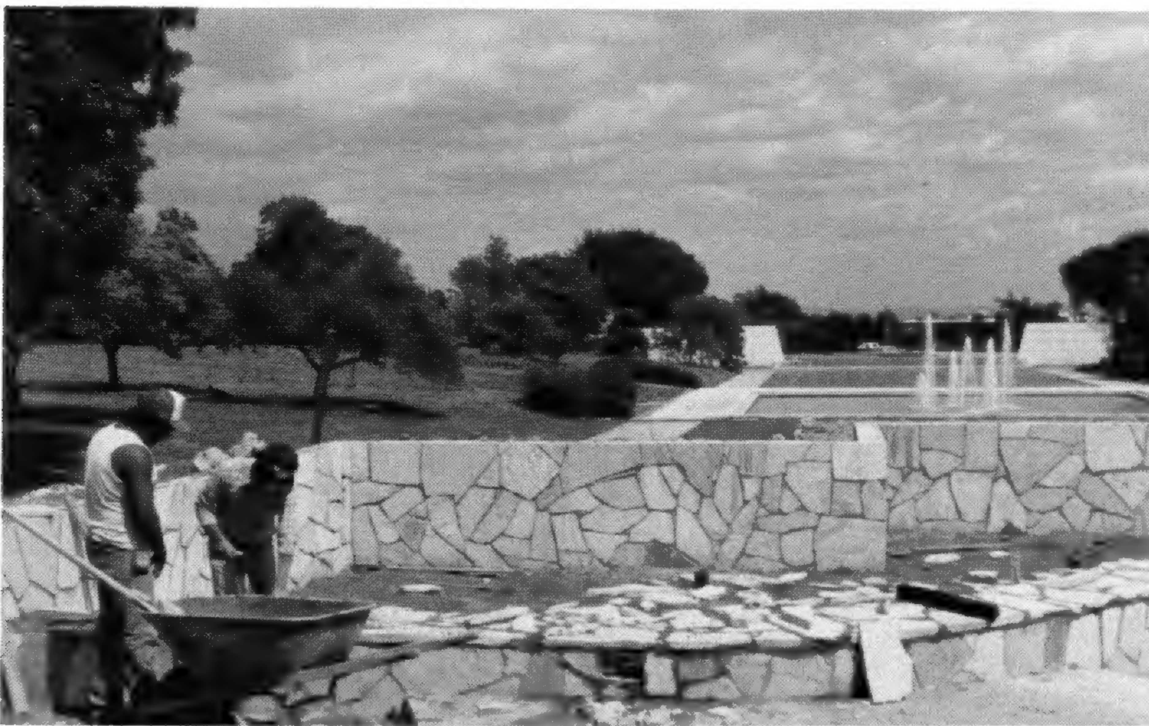
The Drip Wall Bog Garden under construction.
