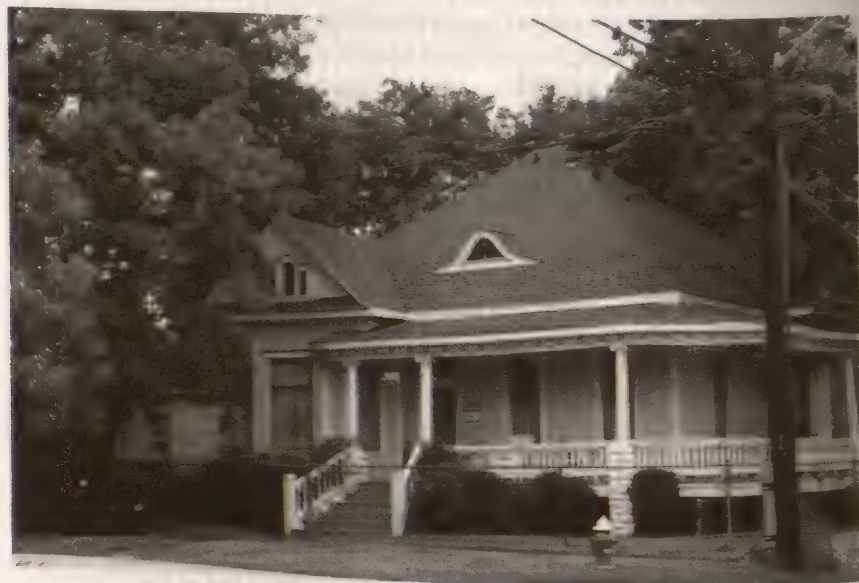
FIGURE 10. A renovated house in the Old Sixth Ward. Photograph courtesy of Shirley Graham.
