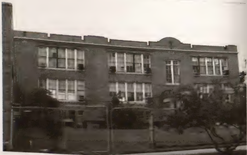
FIGURE 1. Dow Elementary School (unrenovated side). The slide from the third floor extended from the row of windows on the left. Photograph courtesy of Shirley Graham.
