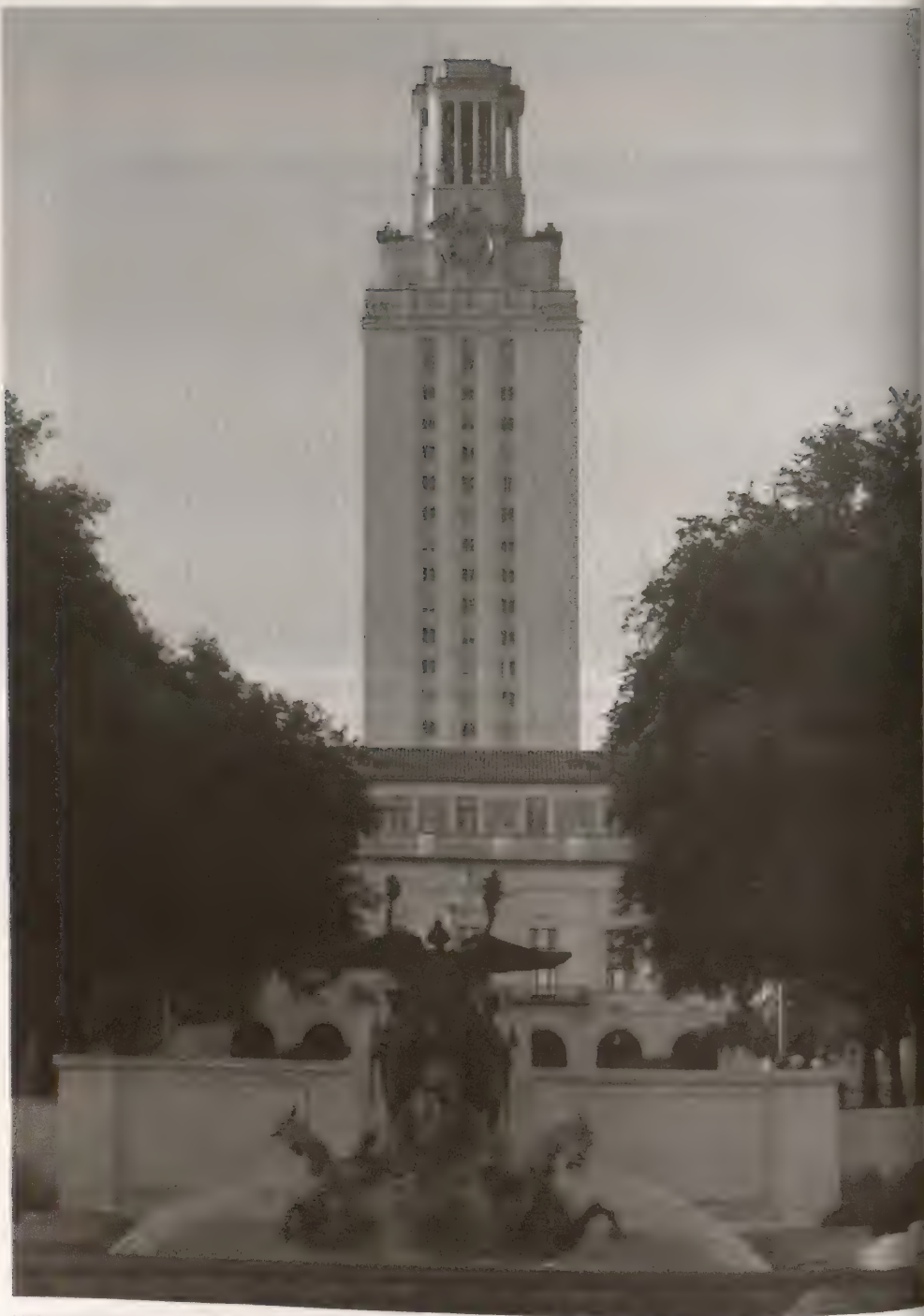
University of Texas Tower, Austin. Photograph courtesy of Tom Wendt.
