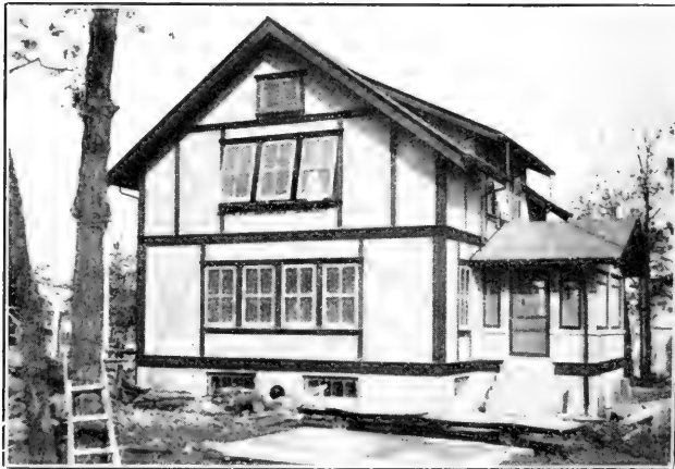
United States Government House for Dam Tender, Gull Lake Dam, 10 miles from nearest town Brainerd, Minn.
