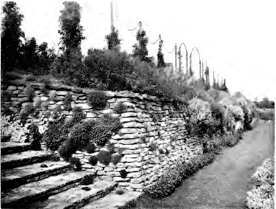
THE NATURAL APPEARANCE OF A ROUGH WALL SHOULD BE RETAINED AT ALL COSTS, SO ONLY PLANTS SHOULD BE CHOSEN THAT ARE SUITABLE
