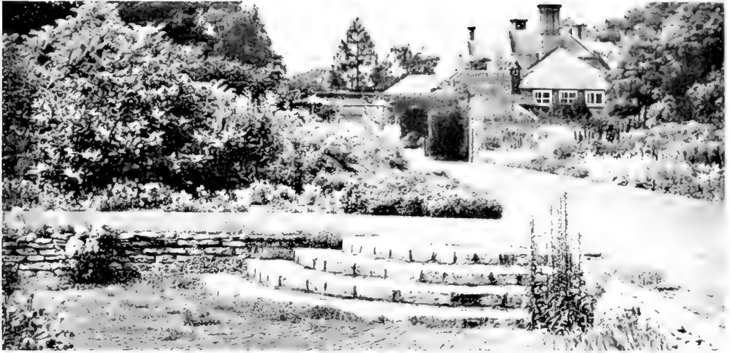
ROUGH STONE STEPS OF CONSIDERABLE WIDTH MAY BE USED IN CONJUNCTION WITH A LOW RETAINING WALL—
