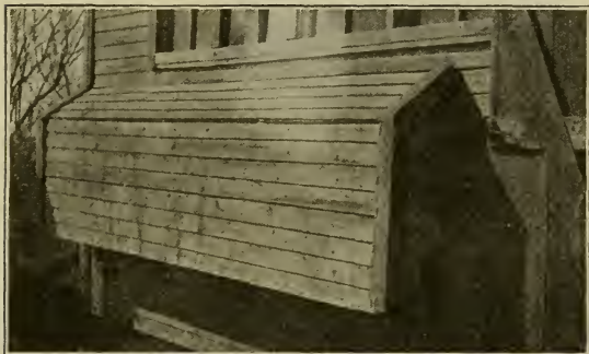
Fig. 30—One Method of Nest Construction to Save Space on Inside of Laying House.
