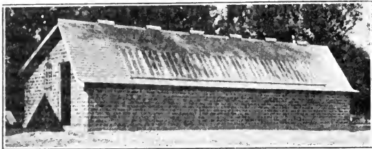
Fig. 6—A Farm Poultry House Built of Hollow Building Tile with Full Monitor Roof.
