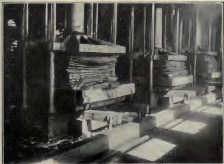
Presses: Barren Island Garbage Reduction Plant.
