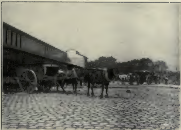
Paris—An Incinerator. Mixed house refuse is brought in large carts and dumped under the shed at the left. It is there picked over and useful articles recovered. The residue is ground up and shipped by rail to the country or burned in an incinerator. The incinerators were new in 1907.
