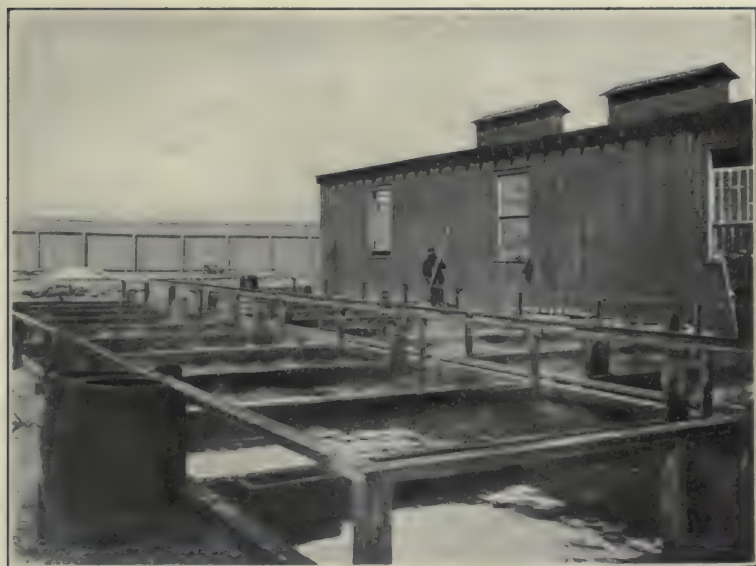
Grease Basins: Barren Island Reduction Plant.
