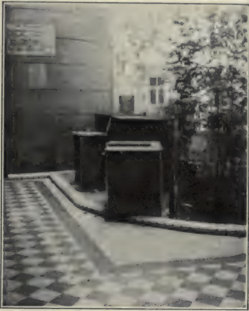
Charlottenburg, near Berlin—Receptacles for the Separate Collection of Kitchen Waste, Ashes, and Paper after, a plan which is a great improvement over that followed in New York.
