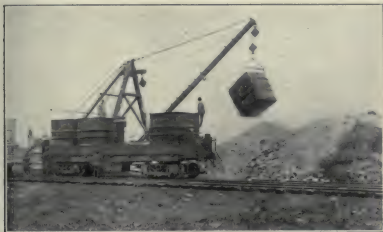
Brooklyn Rapid Transit Ash Dumping Station.
