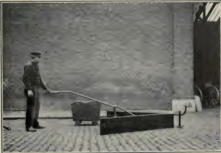
Antwerp—Snow Plough. Low boxes for household refuse fitted together on wheels, in the background.
