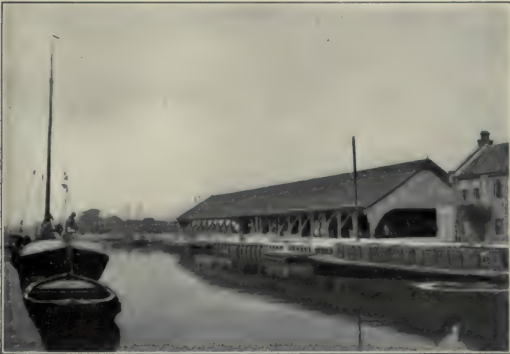
Amsterdam—Refuse Disposal Plant. Picking sheds to the right. Boats loaded with excrement receptacles from dwellings not connected with a sewerage system.
