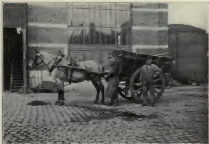
Brussels—Refuse Cart in front of Incinerator.
