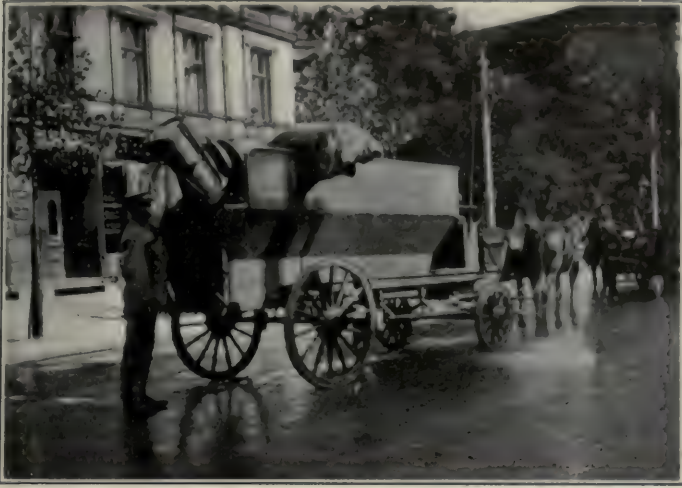
Charlottenburg, near Berlin—House Refuse Cart with Can of Refuse being emptied by mechanical appliance which prevents the escape of dust and odor.
