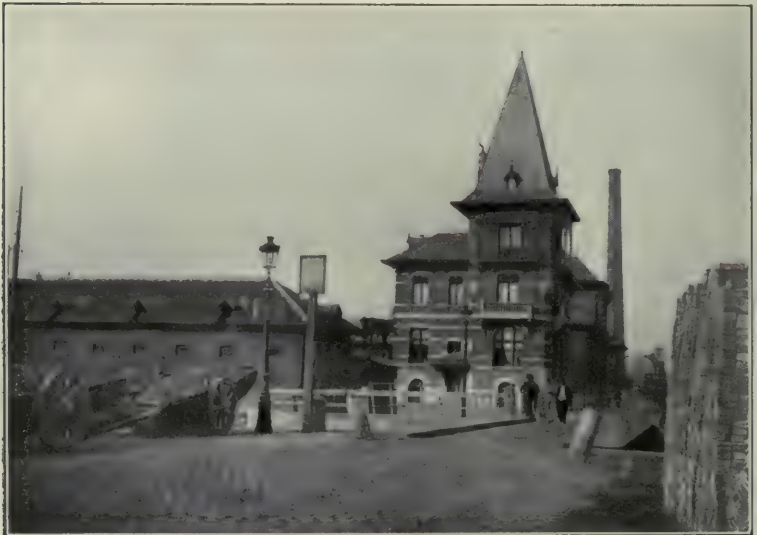
Brussels—Headquarters of Street Cleaning Department. Stack of new incinerator in background. This incinerator resembles the one at Hamburg.
