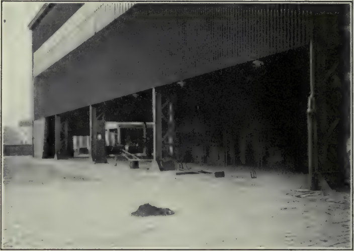
Brussels—Refuse Incinerator. Entrance for teams. Showing the cells where the refuse is burned.
