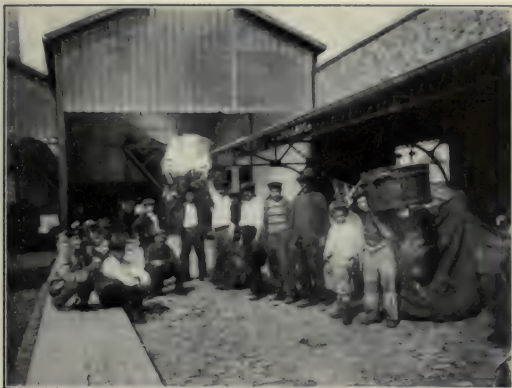
Paris—A Group of Rag-pickers at an Incinerating Plant.
