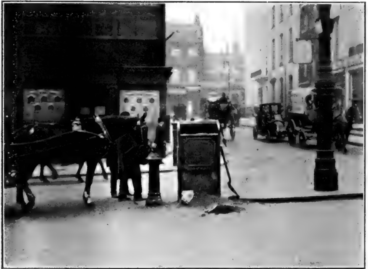
Westminster Sand Bin filled for use. Street refuse is shoveled into a compartment at the top.
