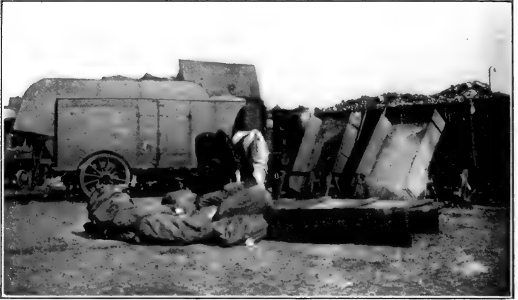
Berlin—Covered Wooden Cart ready to unload refuse upon railway cars for transportation to country for final disposition.
