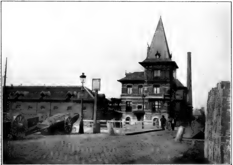
Brussels—Headquarters of Street Cleaning Department. Stack of new incinerator in background. This incinerator resembles the one at Hamburg.
