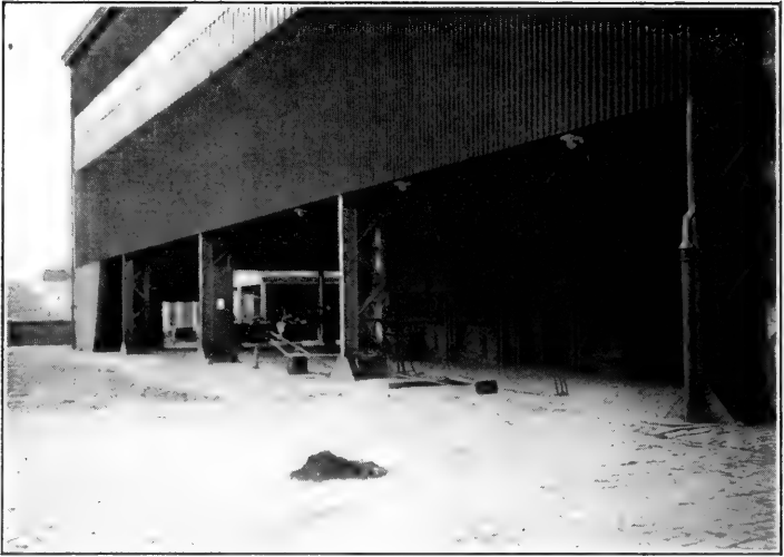
Brussels—Refuse Incinerator. Entrance for teams. Showing the cells where the refuse is burned.
