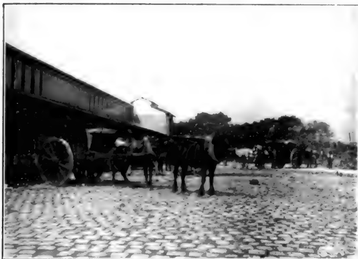
Paris—An Incinerator. Mixed house refuse is brought in large carts and dumped under the shed at the left. It is there picked over and useful articles recovered. The residue is ground up and shipped by rail to the country or burned in an incinerator. The incinerators were new in 1907.
