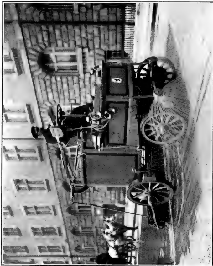
Electrically-driven Machine used in Berlin for Cleaning Streets—the highest development which street-cleaning machines have thus far attained.
