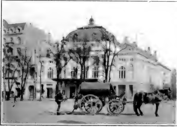
Hamburg—Sprinkling-cart taking Water from a Hydrant placed beneath the pavement.
