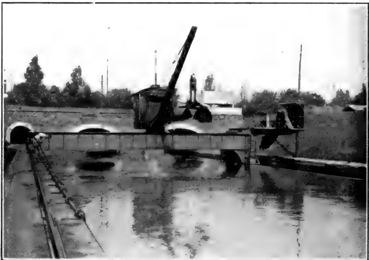
Clichy, near Paris—Settling-basin for the Sewage of Paris. Sand and other heavy, coarse matters settle and are screened here. The basin is constantly dredged. The material excavated is deposited in barges and carried to the country and spread upon land.
