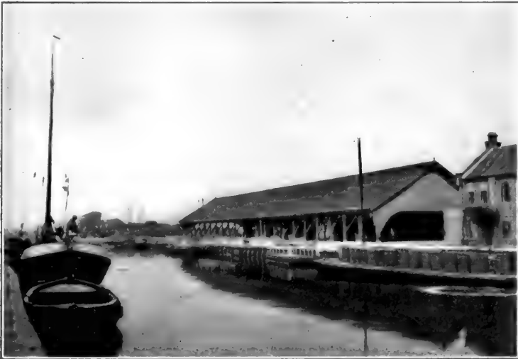
Amsterdam—Refuse Disposal Plant. Picking sheds to the right. Boats loaded with excrement receptacles from dwellings not connected with a sewerage system.
