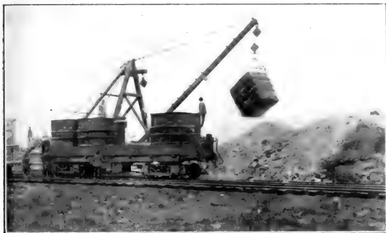
Brooklyn Rapid Transit Ash Dumping Station.
