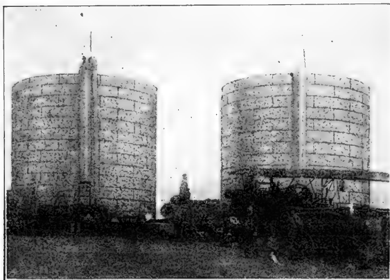
Fig. 45.—Two large Metal Silos and Ohio Cutter at Wagner Bros., Groom, Texas.—Courtesy Perfection Metal Silo Co., Topeka, Kansas.
