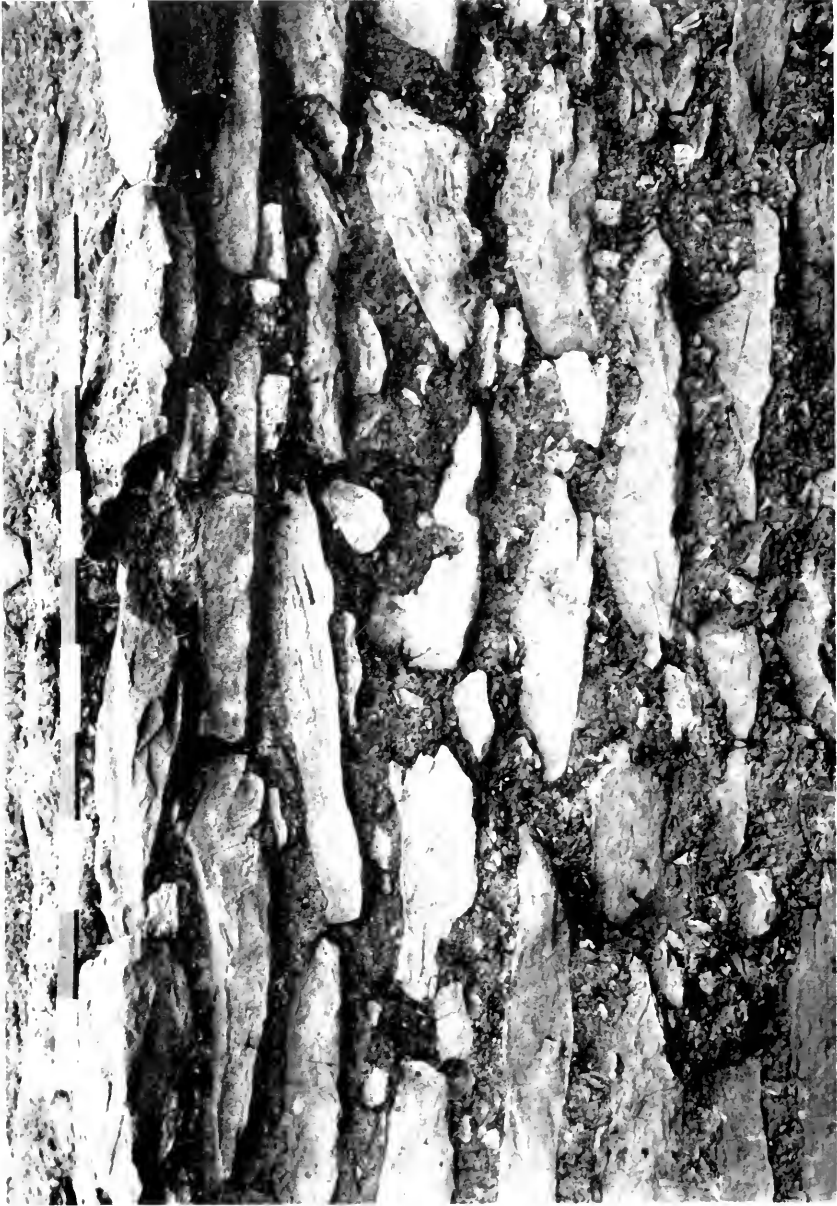
FIG. 67. Site 1, House Group II. Through-stone masonry, north wall, Room 10. Meter stick on top of wall.
