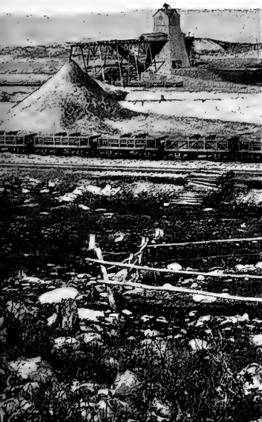
SHAFTS OF THE CHANDLER AND THE PIONEER MINE by open cuts, which have been subsequently enlarged by caving.
