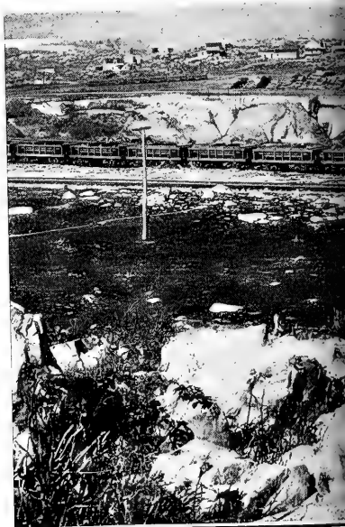
PANORAMIC VIEW OF THE ORE BASIN NORTH OF ELY In the center of the picture is seen the great open pit, caused by
