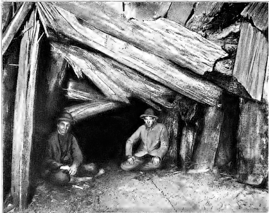
B. VIEW OF MAIN DRIFT WHICH HAS BEGUN TO CAVE, CHANDLER MINE
