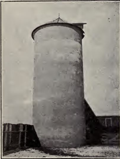
Ed John's Concrete Silo, 16x40 feet, La Fox, Ill. Built by Polk System. W. H. Warford Contractor.
