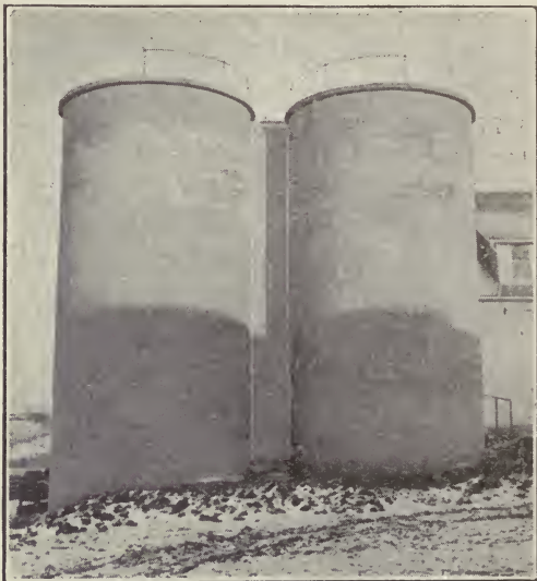
Twin Concrete Silos on farm of Frank White, La Fox, Ill., each 18x45 feet. Built by Polk System. W. H. Warford, Geneva, Ill., Contractor.
