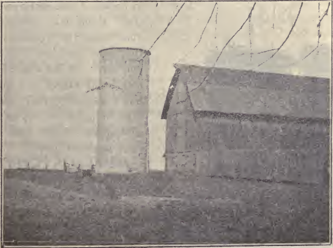
Silo of Mr. C. W. Broughton, McGirr, Ill., diameter 16 feet, height 45 feet. Built by Polk System.
