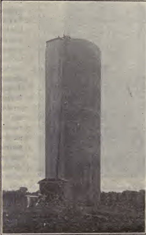
16 x 50 feet monolithic silo of State Hospital Farm No. 1, Fulton, Missouri, showing cutter in position for filling. Built by Polk System.
