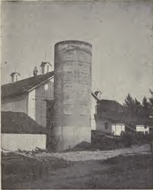
C. M. Saxby's Concrete Silo, Freeport, Ill., 16x40 feet, capacity 1600 tons. Built by Polk System.
