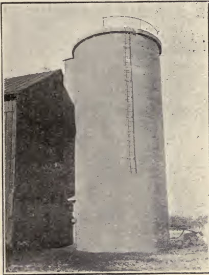
C. A. Baber's Monolithic Silo, LaFox, Illinois. Diameter 18 feet, height 45 feet. Polk System. W. H. Warford, Geneva, Illinois, Contractor.
