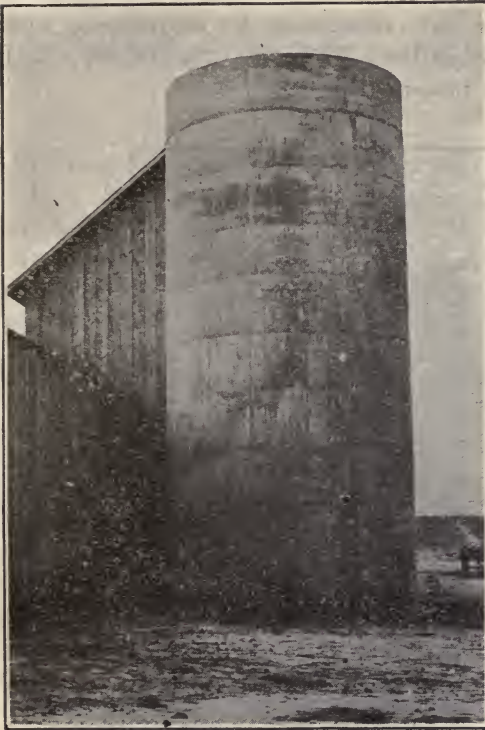
Silo of George Dick, Sycamore, Ill., Size: Diameter 16 feet, Height 40 feet. Polk System
