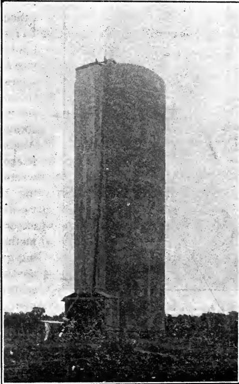
16 x 50 feet monolithic silo of State Hospital Farm No. 1, Fulton, Missouri, showing cutter in position for filling. Built by Polk System.
