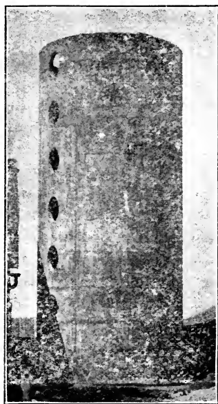
Polk System Silo on George Fox farm, Sycamore, Illinois. Size, 16x40 feet.
