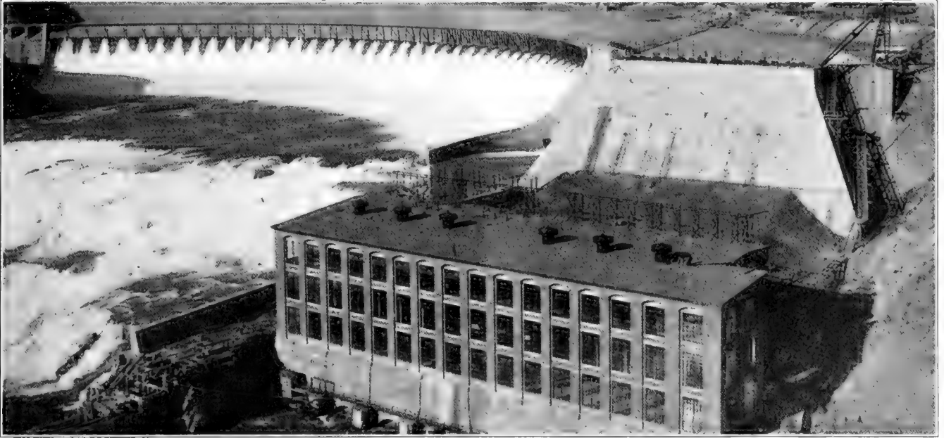
One of a number of Montana Power Company's plants. This one develops 60,000 horsepower
