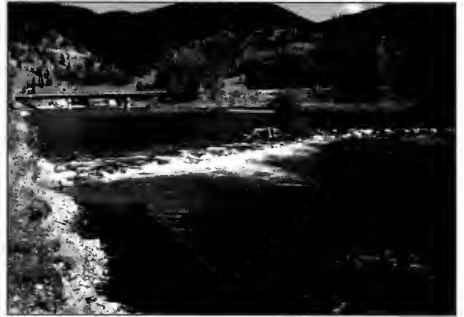
The same structure at left, prior to failure. The warning signs were apparent, notably the elevation of apex above the bed, and 2ft + high drop over the flat sill.
