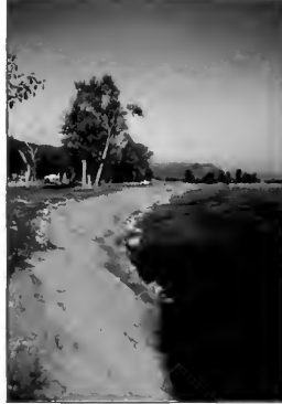
A single wrap of jute mesh fabric with a rock toe provides immediate protection following construction.
