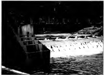
Denil fish ladders should be long enough to ensure that the outlet end is submerged during operation.
