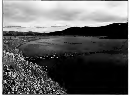
A bendway weir has a gradually sloping profile which shifts the main channel of the river to the outside of the structure. Peak flows continue to use the channel cross section above the weir elevation.
