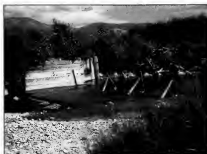
Wooden diversion structures have a limited life but are easily constructed.
