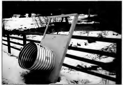
Typical prefabricated metal R-5 headgate structure used for squash or arch pipes.
