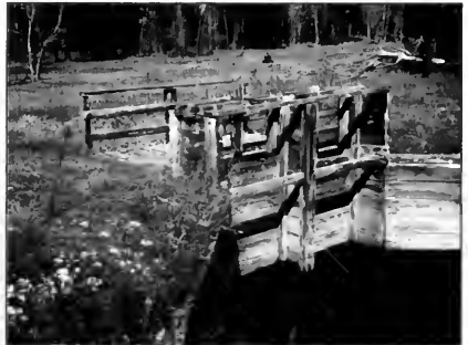
This is a well-constructed gate with wingwalls and positive control at high flows.
