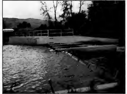
Inflatable bladder gates are generally used in specialized applications where precise control of water is important.
