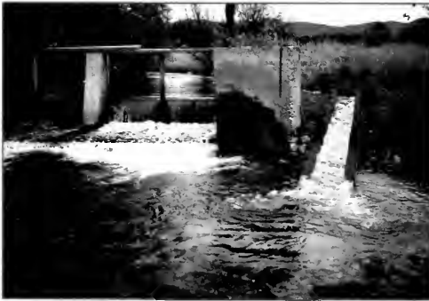
Denil fish ladders have a series of baffles to allow fish passage for small diversions.
