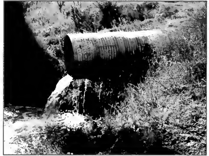
The shotgun (or perched outlet) culvert impedes fish passage, and can result from placing the culvert too high, or installing the culvert in a channel that has a tendency to downcut without grade control downstream of the outlet.
