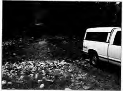
To protect water quality, avoid fords on perennial channels with poor approaches and inadequate drainage control.
