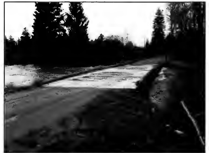
Stream crossings on shallow channels with broad floodplains must rise to meet the bridge, or the bridge will end up being too low, like this one.
