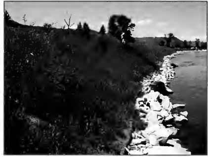
Same bank as above 14 months later. This is essentially a hard stabilization approach because the rock toe makes the stabilized bank stronger than a natural bank.
