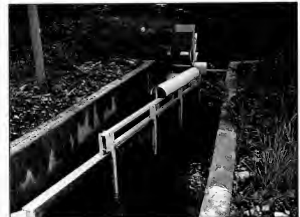
Fish screens are effective for preventing fish loss in irrigation ditches. A by-pass channel is needed to redirect fry to the main channel. A flat screen relies on brushes to clear debris.
