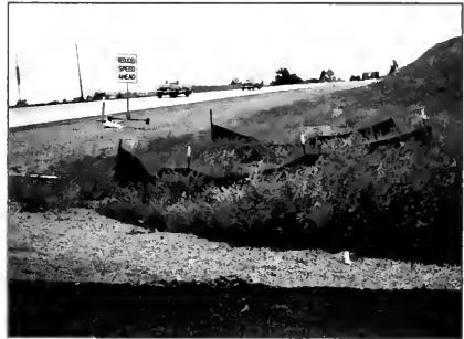
Silt fence helps prevent sediment delivery on newly constructed roads, but does not substitute for proper drainage features.
