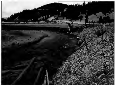
Erosion has moved downstream below this rip-rapped bank.
