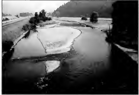
Rip-rap on channelized reaches will limit the ability of the stream to re-establish equilibrium.
