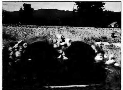
A half-hearted effort at armoring the inlets, but note that the pipes are set below grade, which is good for fish passage.
