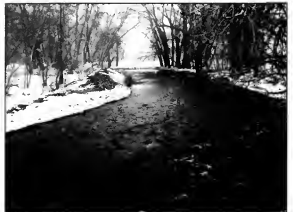
Attempting to control flooding on aggrading channels with excavation and berms is rarely successful because the channel continues to fill.
