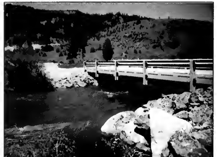
The structural beam on many railcars hangs low and ends up falling below bankfull elevation.
