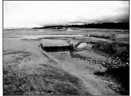
This large concrete structure functions as a cipoletti type weir.
