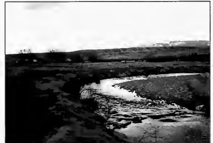
This meander has been restored with channel shaping, grade control structures, root wad/woody debris, and bank sloping sod mats.
