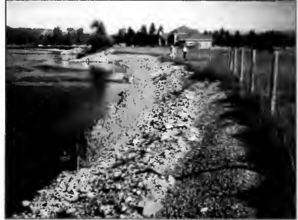
Live willow cuttings seem to survive best when cut and planted in the early spring prior to bud break.
