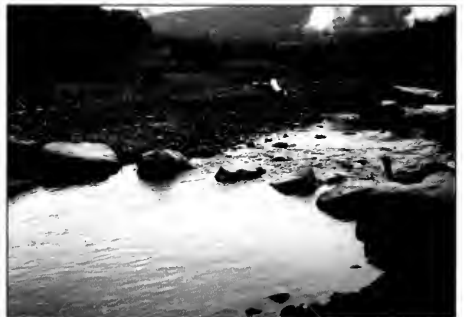
True "V" weirs generally have a row of cap rocks with spaces, rather than a flat sill. This promotes bedload passage (to some extent), but does not always work well for irrigation diversion needs.
