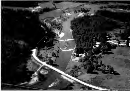
These large weirs eventually failed because they were built too high, and restricted sediment passage.
