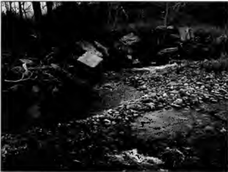
Concrete is generally not acceptable for rip-rap.
