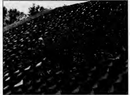
A cellular confinement system can be effective for steep slope stabilization and revegetation.
