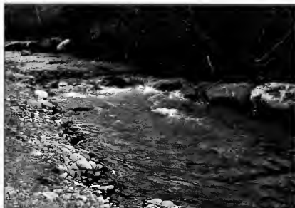
Barbs are constructed with a low sloping profile and gently "roll" the current away from the bank.
