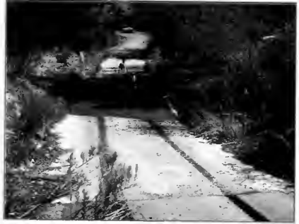
Fords may be a viable alternative for intermittent or shallow wide channels that resist other solutions.
