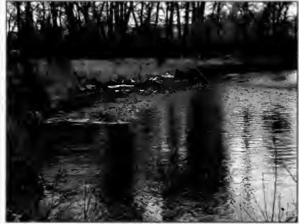
Four years later bank remains stable at this site. Three short low profile barbs were used to reduce near-bank velocities.
