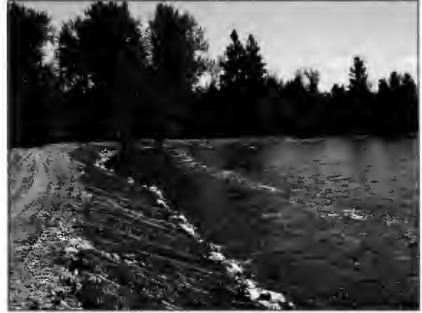
This levee was stabilized to protect downstream development from flooding, although the landowner with the levee did not particularly want to constrain the river.
