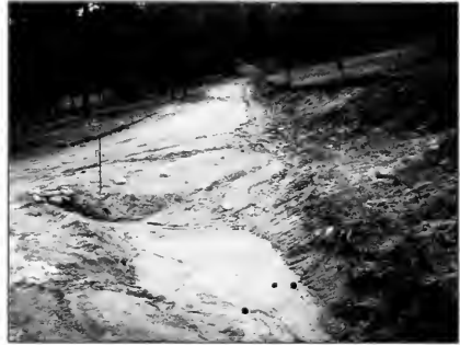
Poor drainage on granitic soils can deliver large amounts of sediment to streams.
