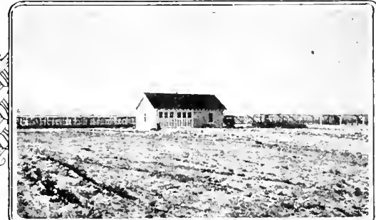
FEED ROOMS AND GARAGE WITH PENS IN BACKGROUND
