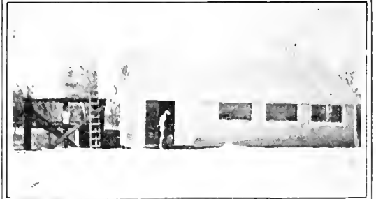
TANK HOUSE—LAKE GARBERTSON.
