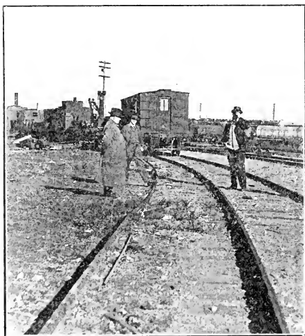
FIG. 105.—Spur track and steam pipe line used for disinfecting cotton cars. (Photo by L. A. Whitney.)
