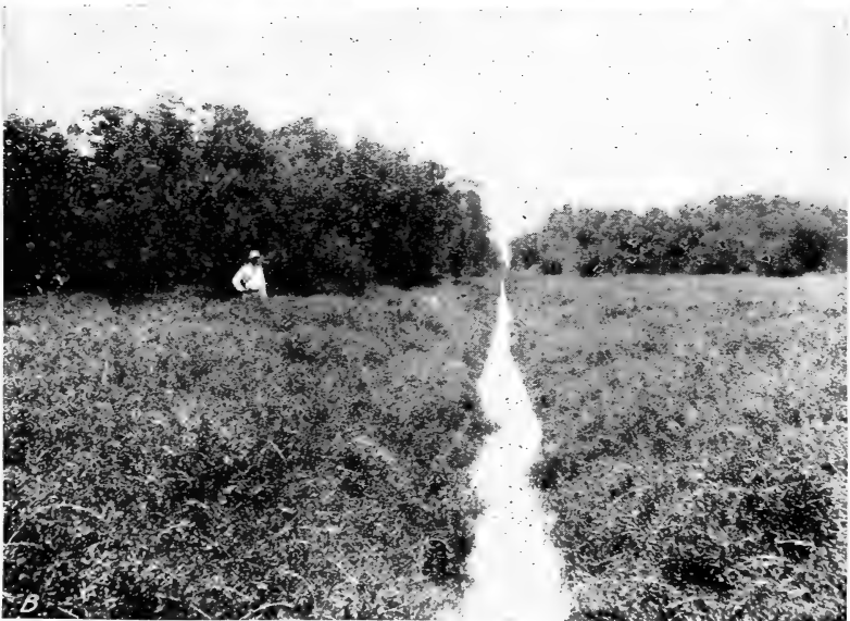
Mosquito-control ditches in salt-marsh areas: A , In North Carolina; B , in Florida, pickleweed in foreground, mangrove trees in background.
