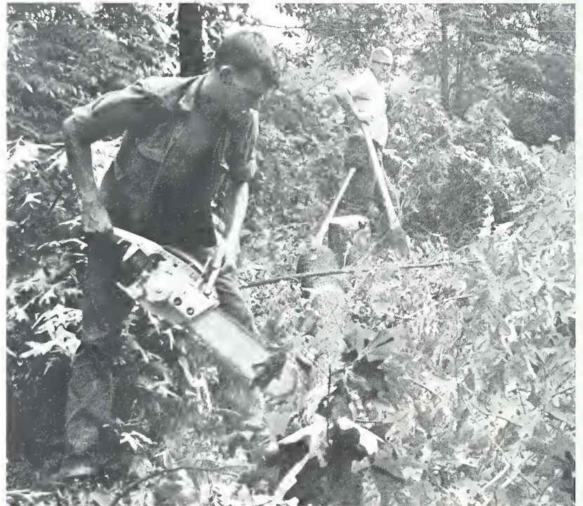
Clearing out for the new building.
