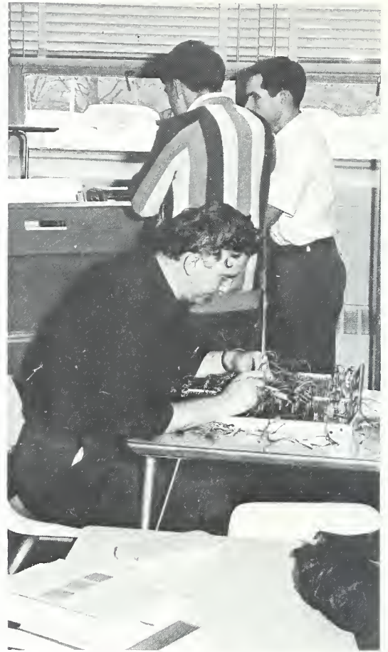
Wiring a panel.
