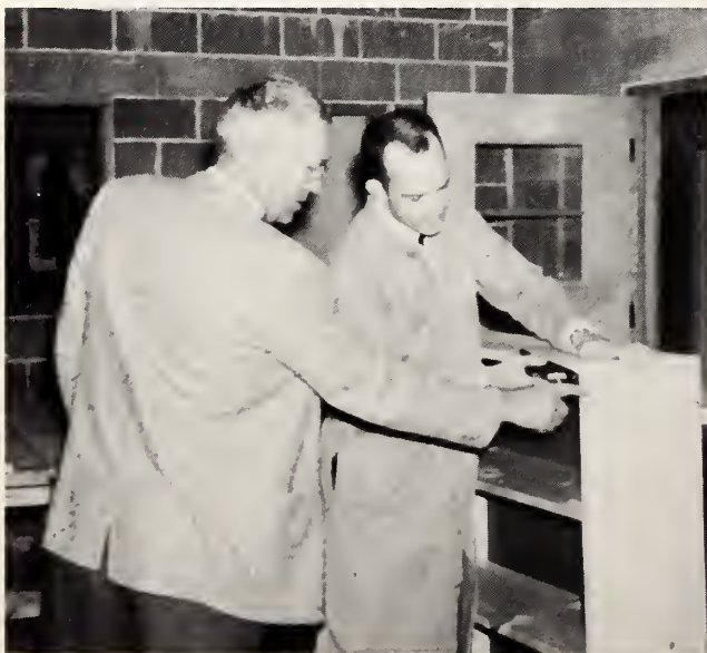
Carpentry in the new unit.
