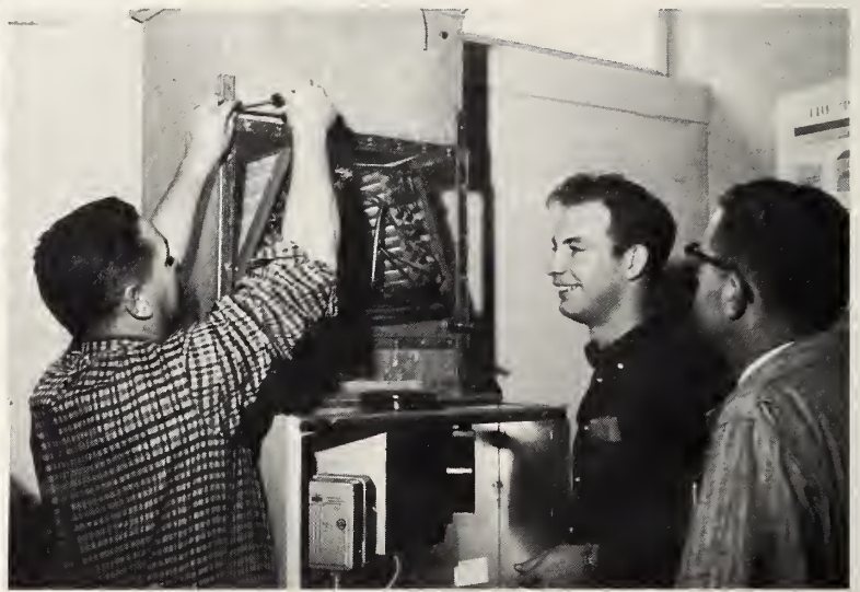
Installing an inspection panel.
