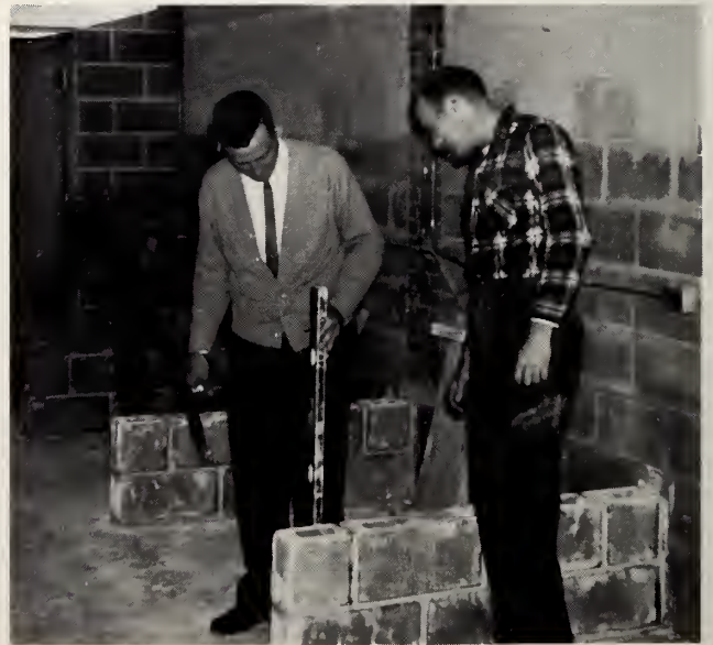
Brick Laying at Sylva
