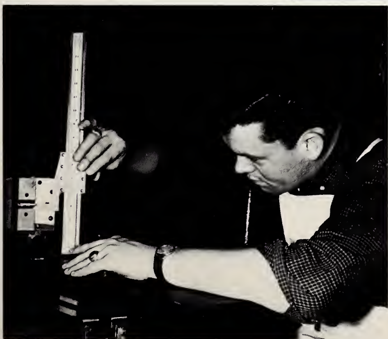
Measuring with height gage.
