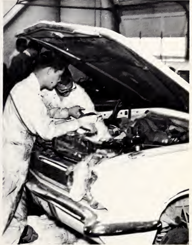
Installing Shocks and Relining Brakes
