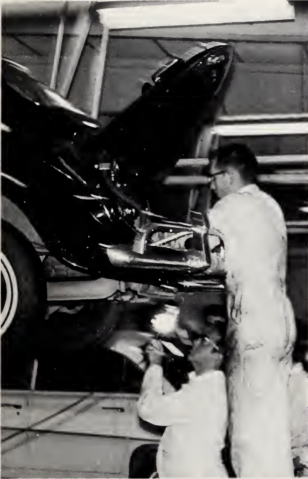
Replacing the Engine in a Volkswagen
