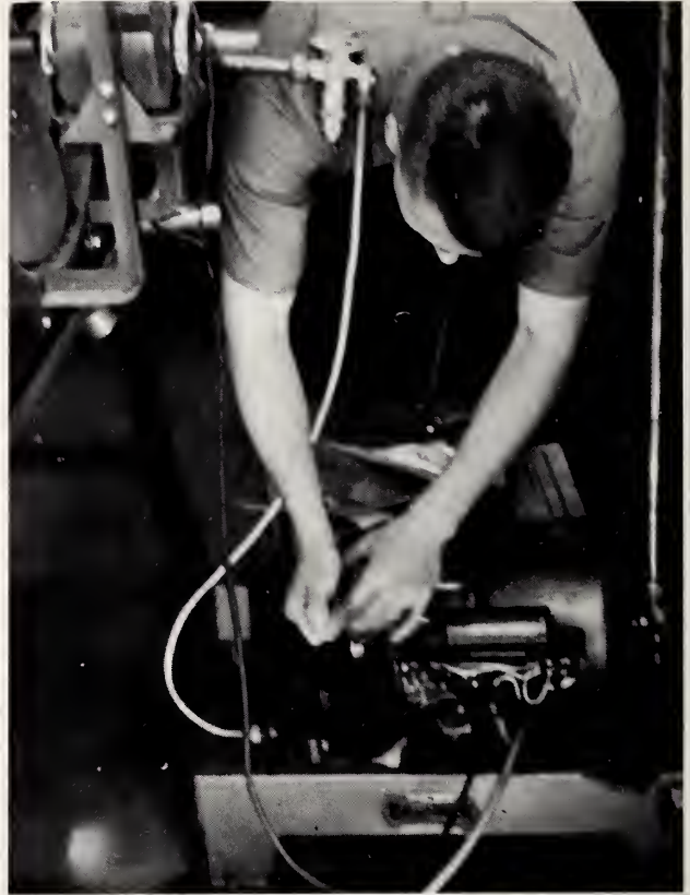
Installing a Condenser Unit
