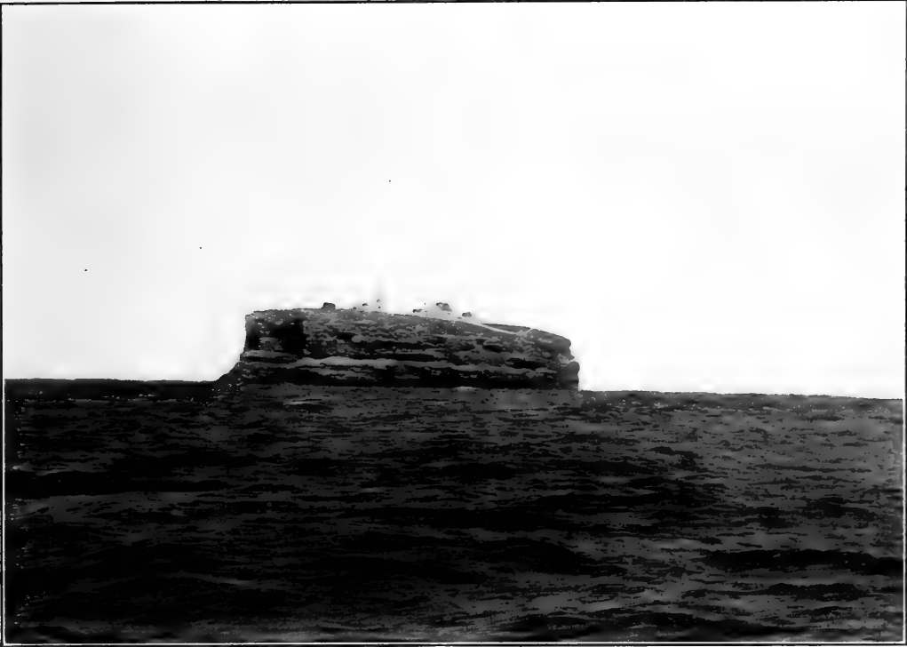
Great Bird rock, from the south; showing light house and accessory buildings
