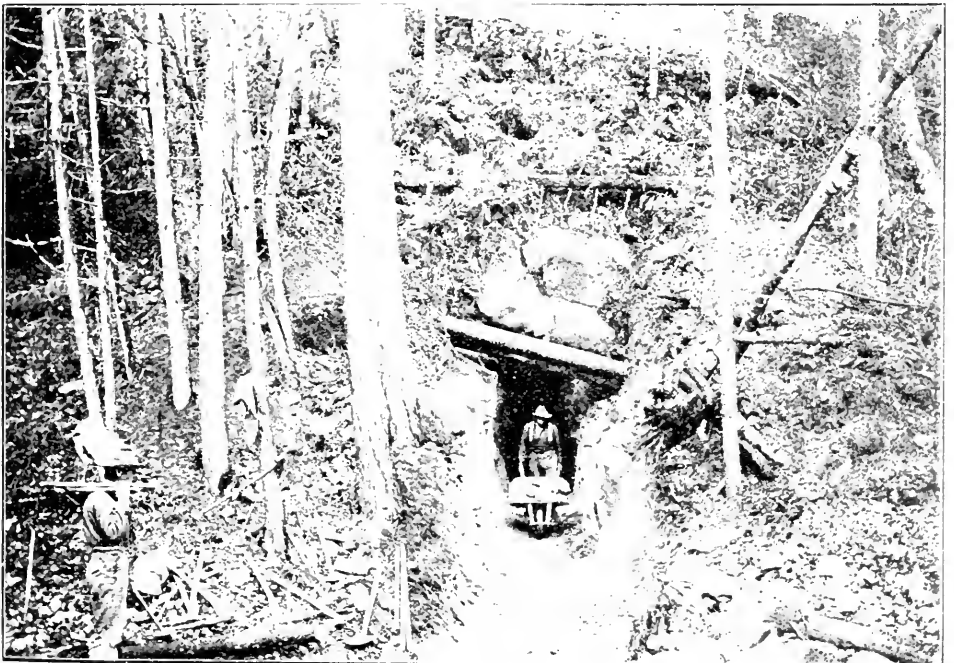
5. Tunnel of Gold Sun Mine, Gray Lake, p. 1.
