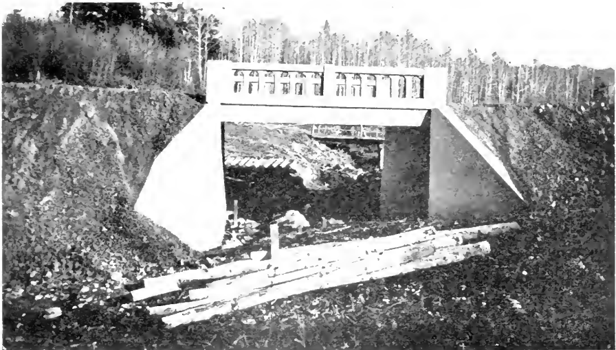
Stoney Creek bridge—International Highway.
