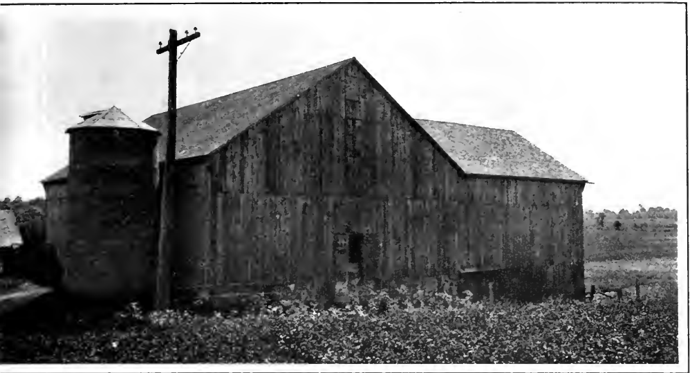
SERVICE IN ONTARIO Ontario, using "Hydro" service
