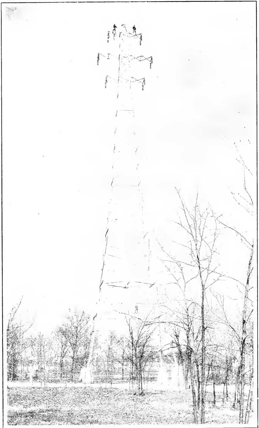
EASTERN ONTARIO HIGH-VOLTAGE TRANSMISSION LINES Ottawa River crossing towers nearing completion. Note figures of men
