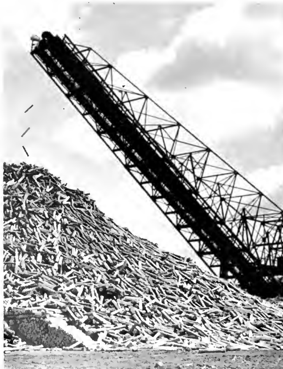
BUILDING PULPWOOD RESERVE PILE AT MILL
