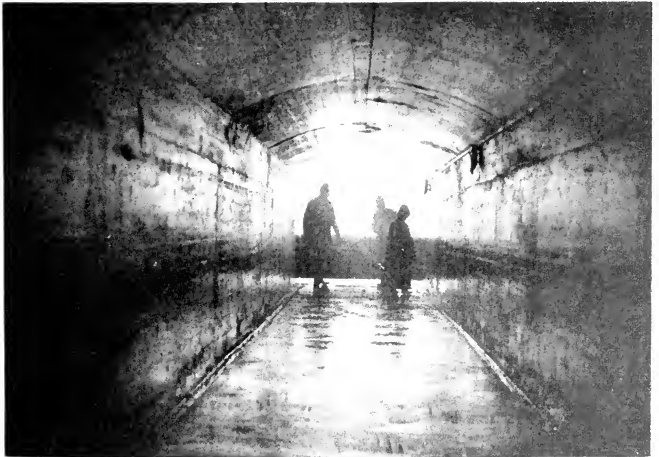
Part of New Table Rock Tunnel Beneath Horseshoe Falls
