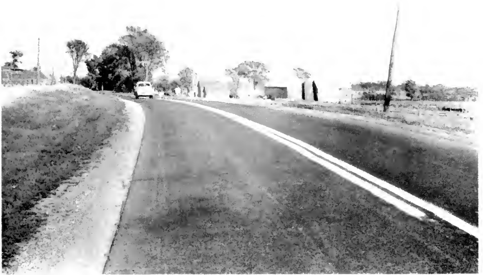
Double solid lines indicate crossing from either side is prohibited.
