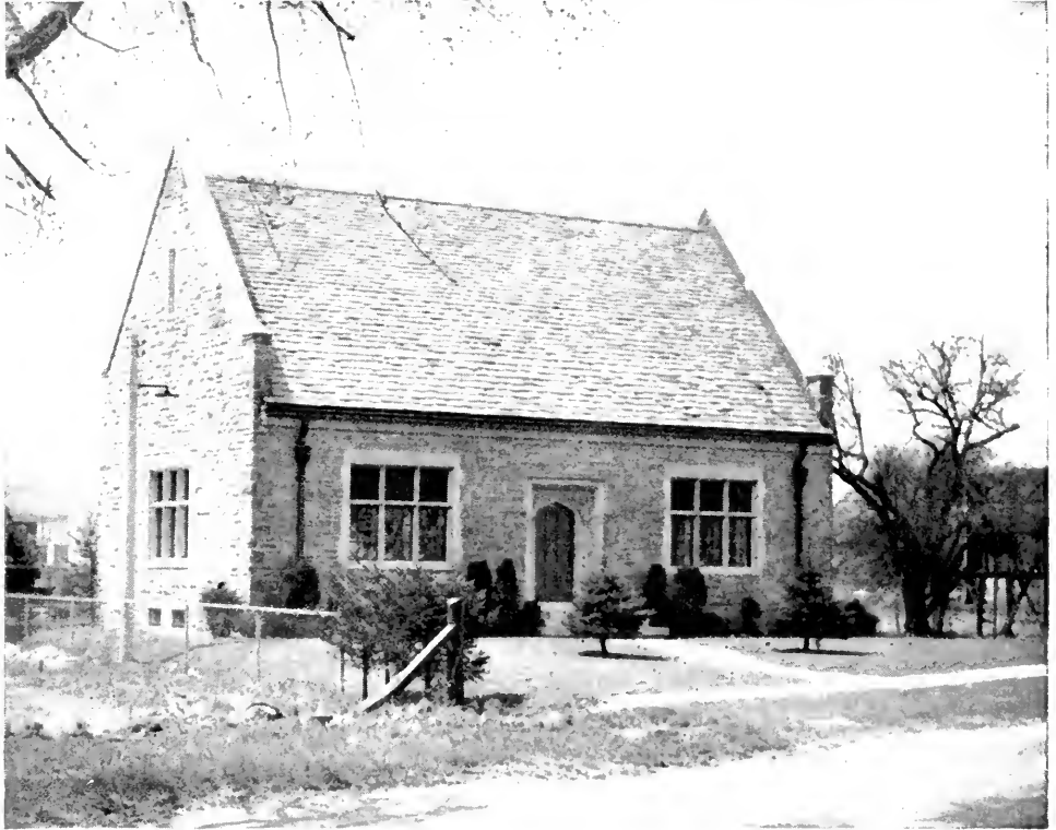
A Hydro substation in keeping with its residential environment. Strouds Lane, Hamilton
