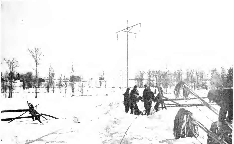
LINE CONSTRUCTION IN THE WINTER
