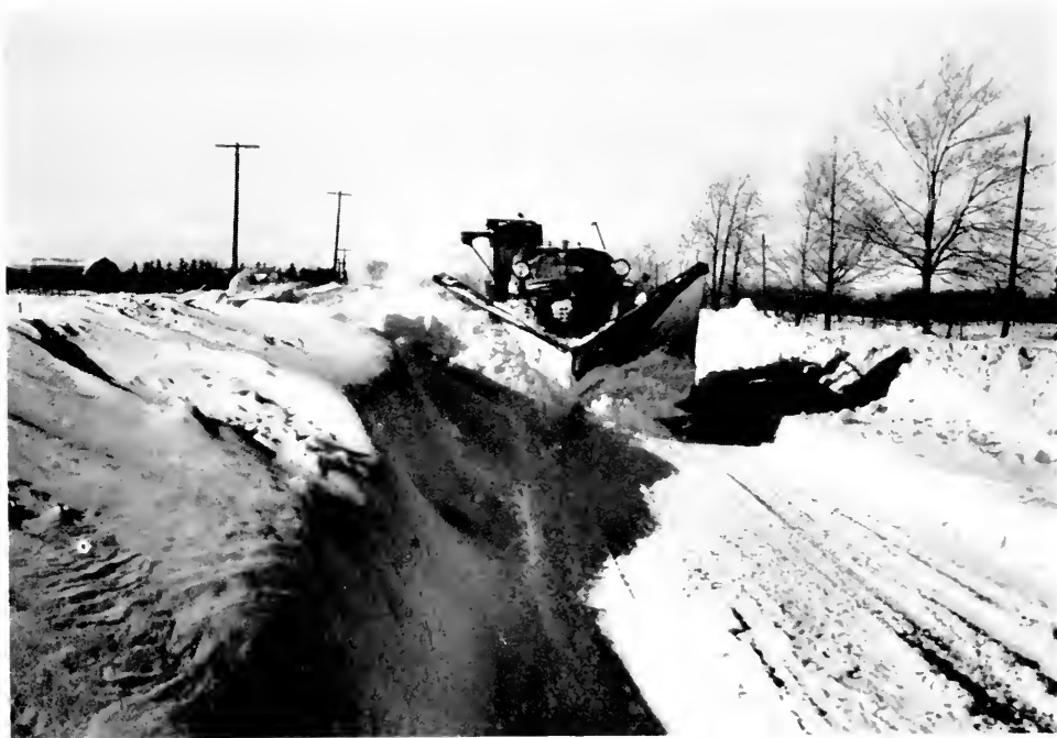
V-plow widening highway in Niagara Peninsula.
