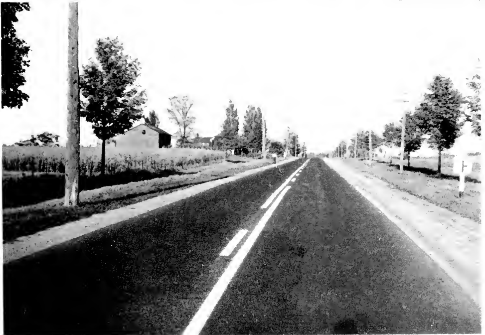
On double markings, when solid line is on your side, crossing of same is prohibited; if you are on the dotted side you may cross if the way is clear.
