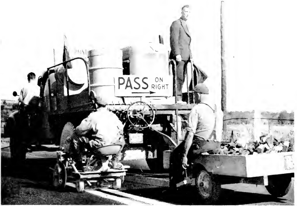
Zone-striping equipment in operation.
