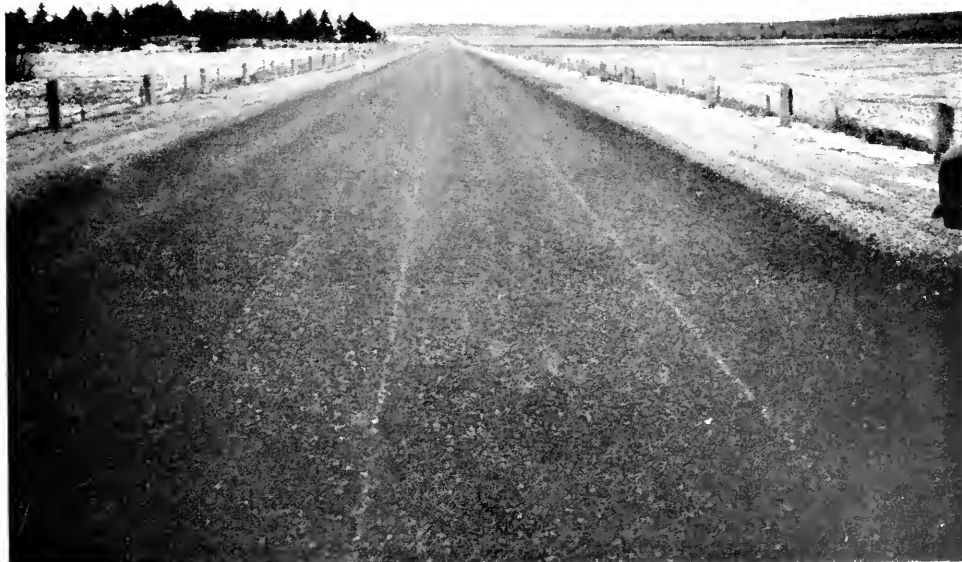
Mulch surface, Highway No. 17, five miles west of Sturgeon Falls
