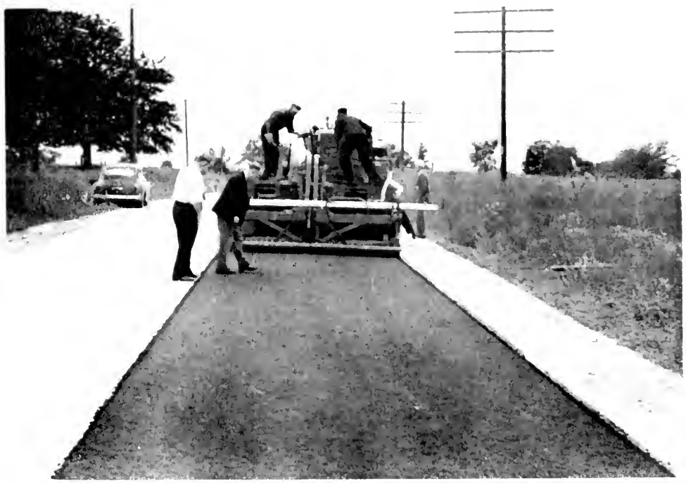
Laying bituminous carpet coat.
