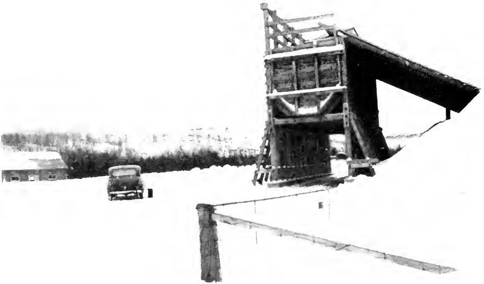
Sand loading bin located at junction of No. 11 Highway and Airport Road near North Bay.
