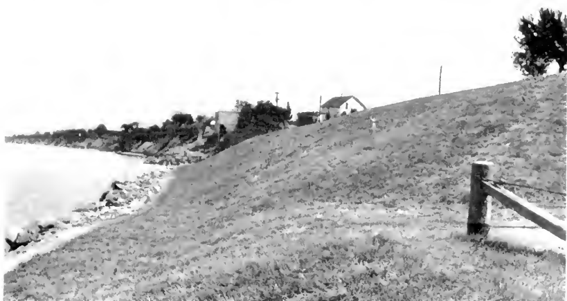
Finished graded and sodded shoreline.
