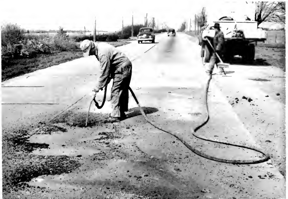
Asphalt jacking operations.
