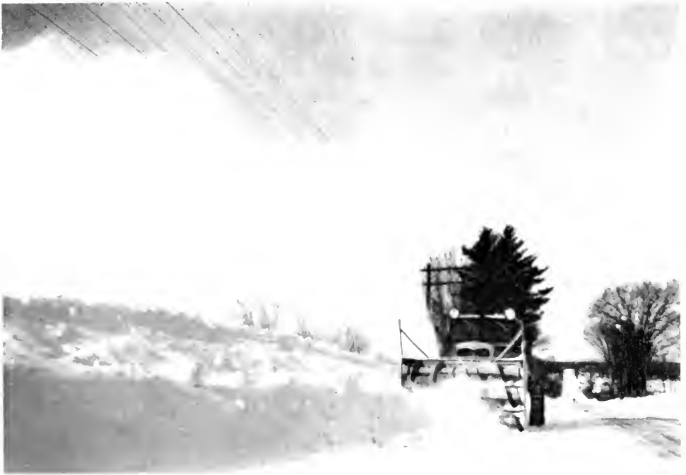
Rotary plow in operation
