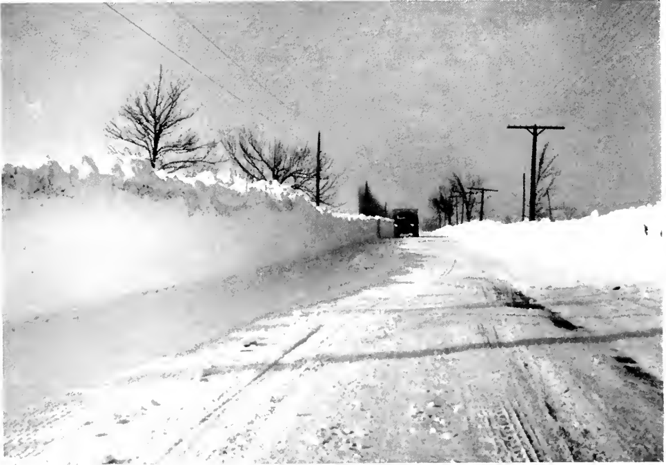
A winter highway widened by rotary plow.
