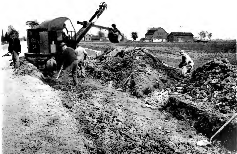
Excavating disintegrated roadbed on Highway No. 3 between Jarvis and Simco
