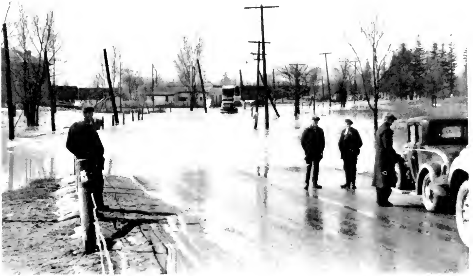
Spring flood conditions on Highway No. 2 at Pickering
