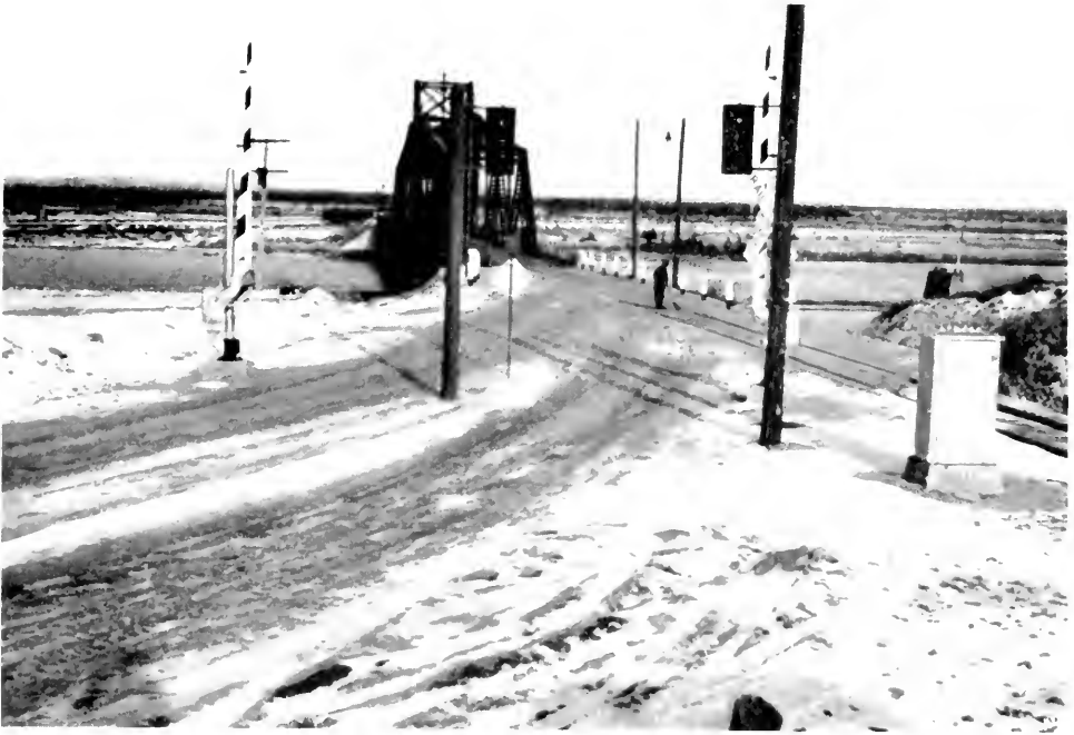
Approach to bridge at Little Current, showing traffic signals to control both train and motor vehicle traffic.
