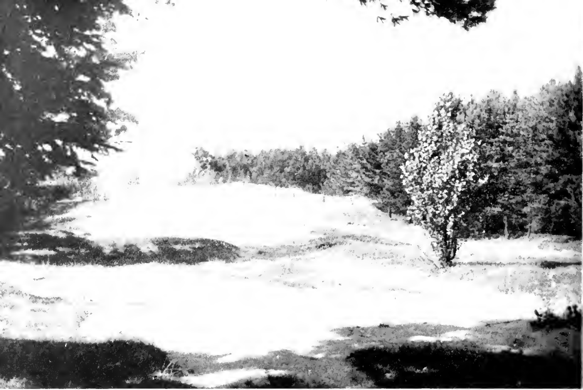
Blow-sand has made this road unfit for use. Note the plantation on the right which is correcting this condition. Ontario County.
