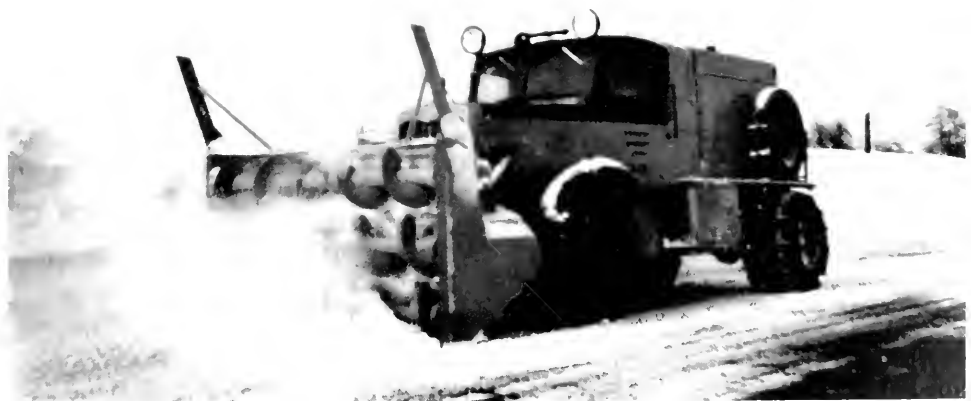
Close-up view of rotary plow in operation.
