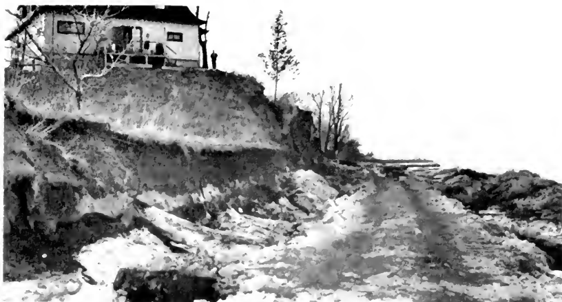
Sea wall under construction to retard erosion of shoreline
