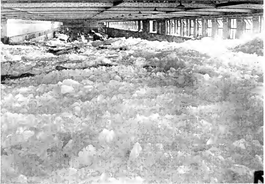
Figure 1—The interior of the powerhouse, facing the down-stream end, after the water had receded
