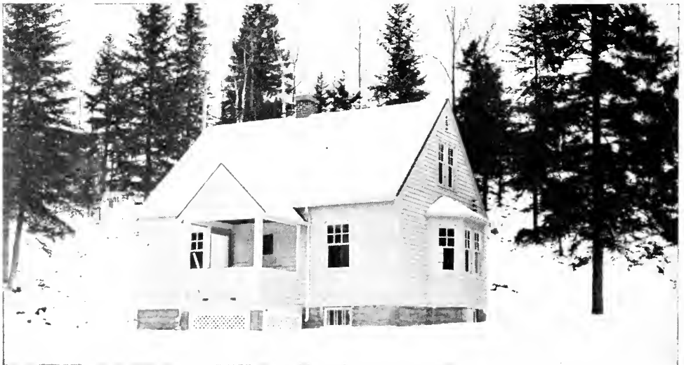
CAMERON FALLS DEVELOPMENT—NIPIGON RIVER Operator's house
