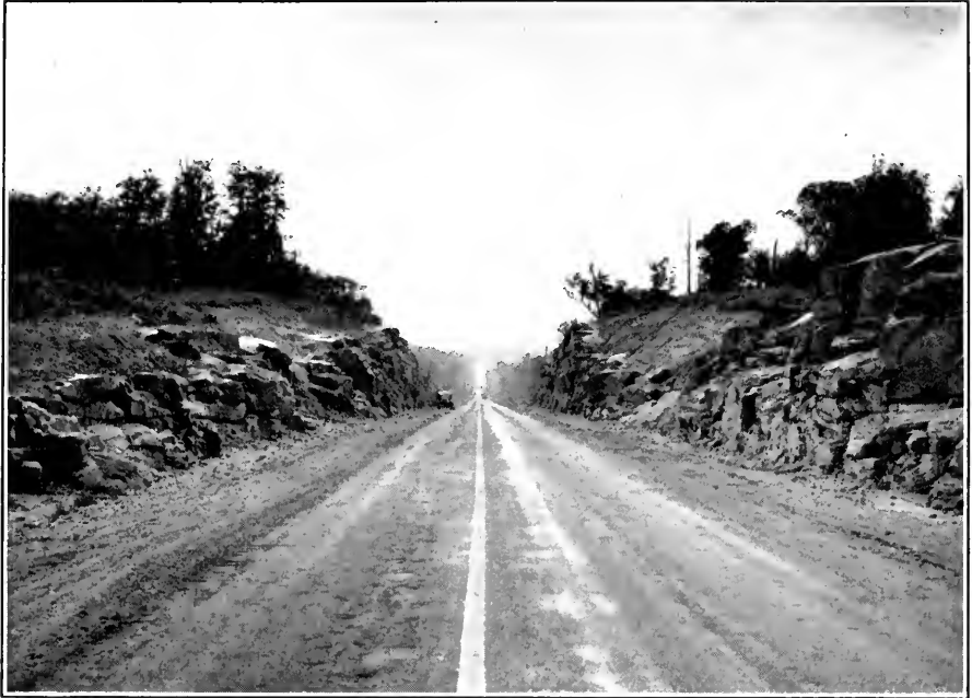
Rock cut and fill south of Powassan, Highway No. 11.
