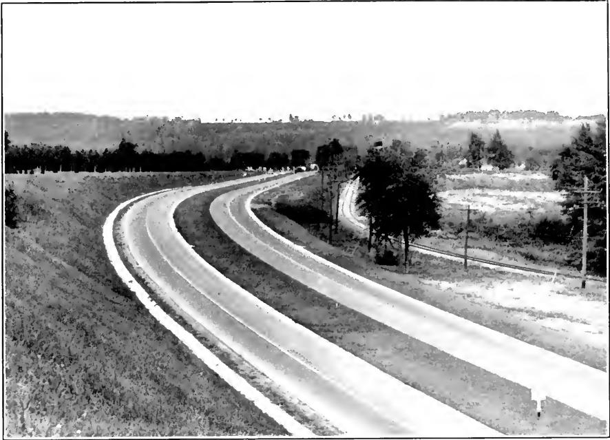
Dundas Diversion, looking toward Hamilton.
