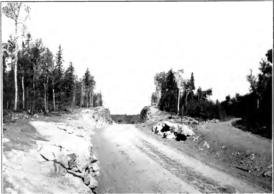
Looking north toward rock cut, north of James Lake, Highway No. 11.
