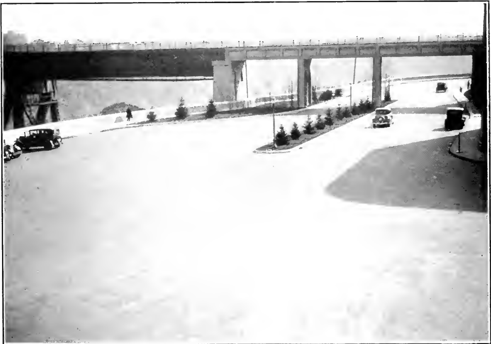
Improvements, vicinity of Lower Arch Bridge—Railway tracks, old buildings removed
