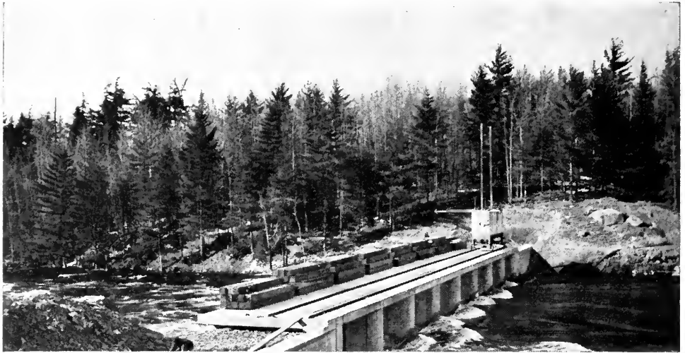
RAGGED RAPIDS DEVELOPMENT—MOON RIVER DAM
