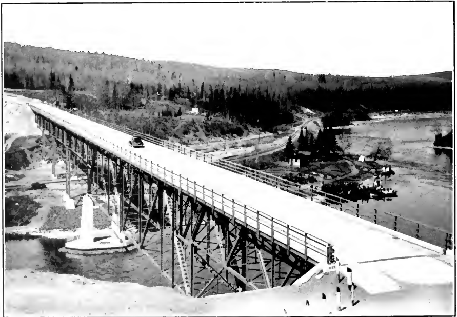
Nipigon River Bridge on Trans-Canada Highway, east of the Village of Nipigon. Total length, 772 feet 8 inches. Centre span, 220 feet.
