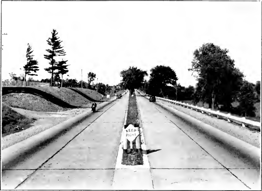
The Middle Road looking east, east of Bronte Bridge.
