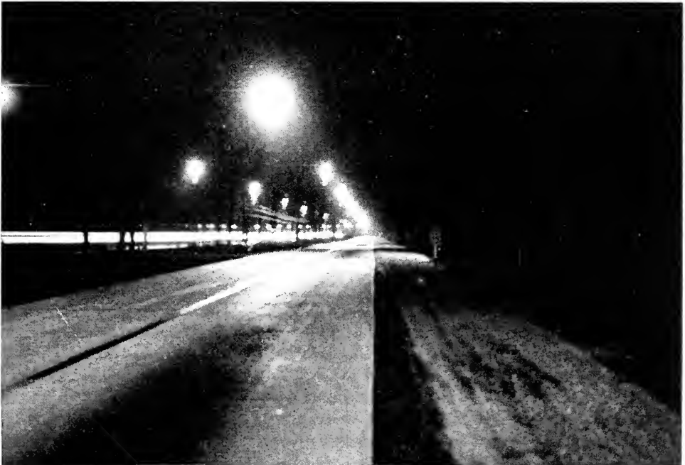
LIGHTING OF DUAL HIGHWAY, TORONTO TO BURLINGTON Night view
