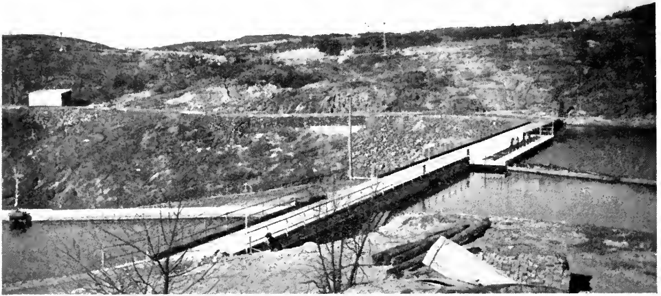
CONISTON DAM — FROM UPSTREAM SIDE
