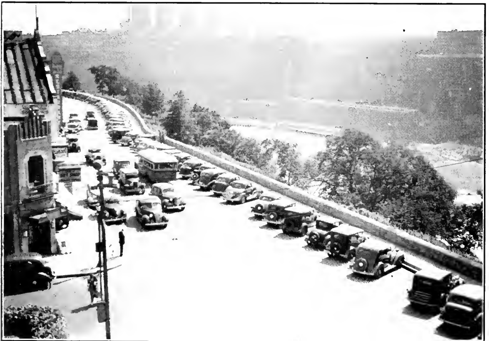
River Road, vicinity of Falls View Bridge
