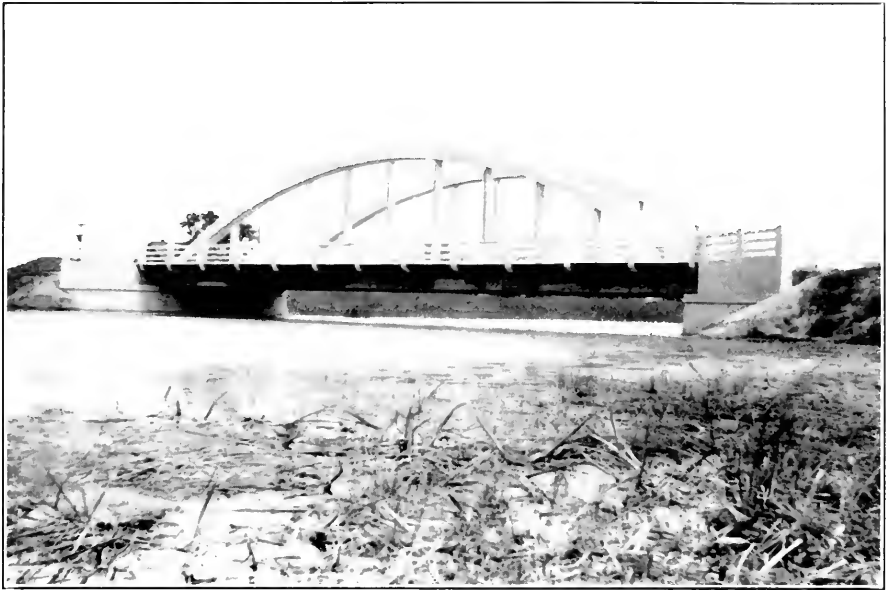
Bridge over River Canard at Loiselleville, Essex County, Road No. 20. Built in 1937; 120-foot span.
