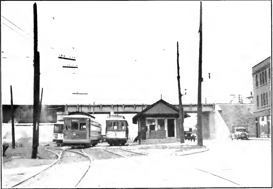
Improvements, vicinity of Lower Arch Bridge—Railway tracks, old buildings, etc., before removal
