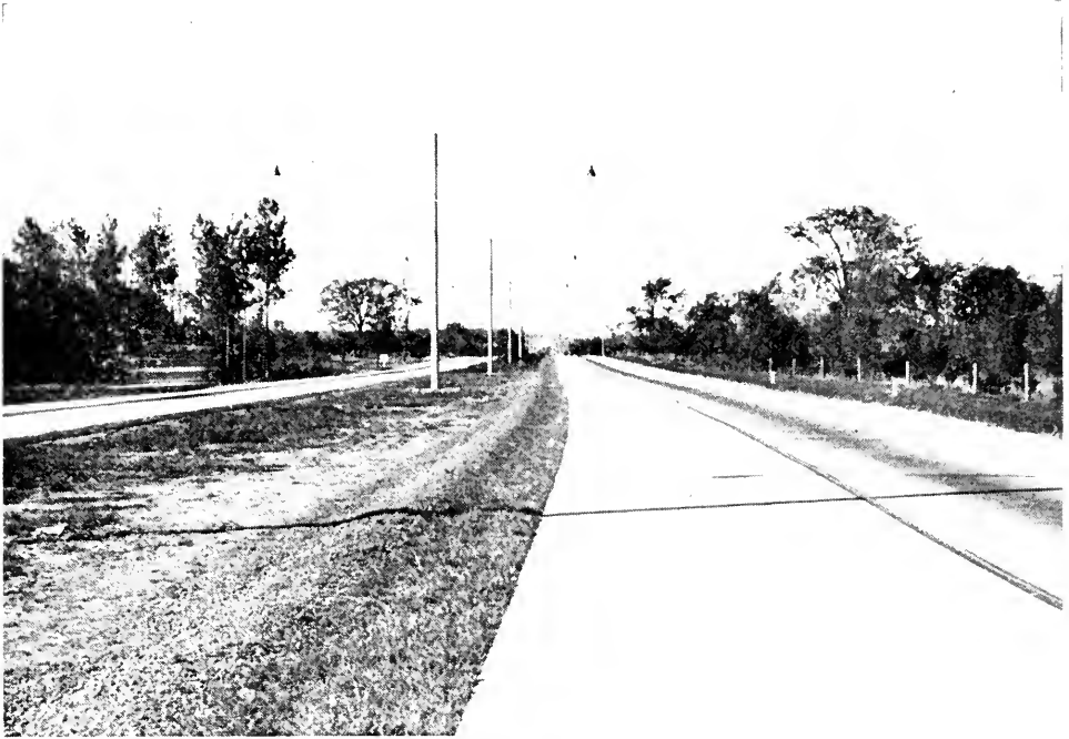
LIGHTING OF DUAL HIGHWAY, TORONTO TO BURLINGTON Supports are placed in centre boulevard, wires are underground
