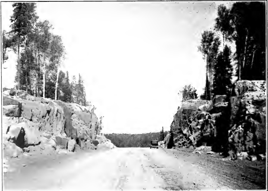
Rock cut, north of James Lake, Highway No. 11.
