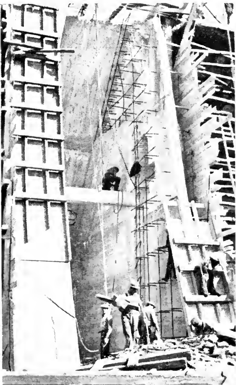
EUGENIA FALLS DAM Repairs to structure by reinforcing piers
