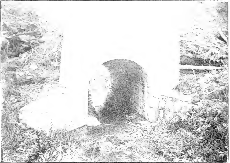
ARCH COVERED OF CONCRETE
