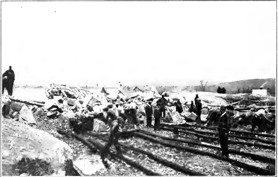
East face of Rock Cut at North Bay.
