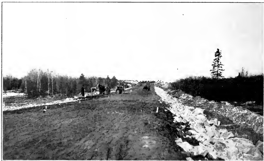
Riprapping grade between Rock Cuts.
