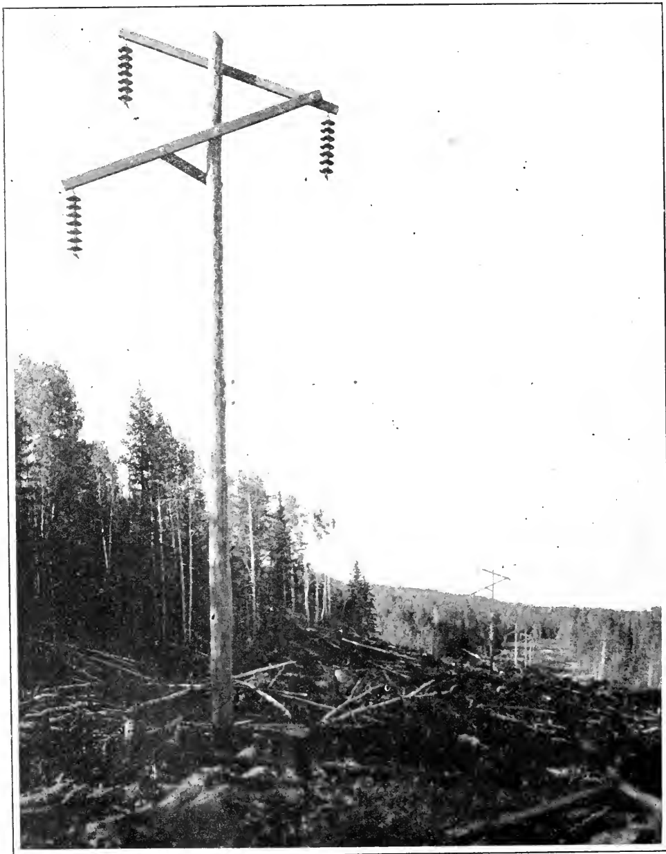
Standard wishbone construction, Nipigon Transmission Line, looking north about three miles to Generating Station. (Ground wire not placed.)
