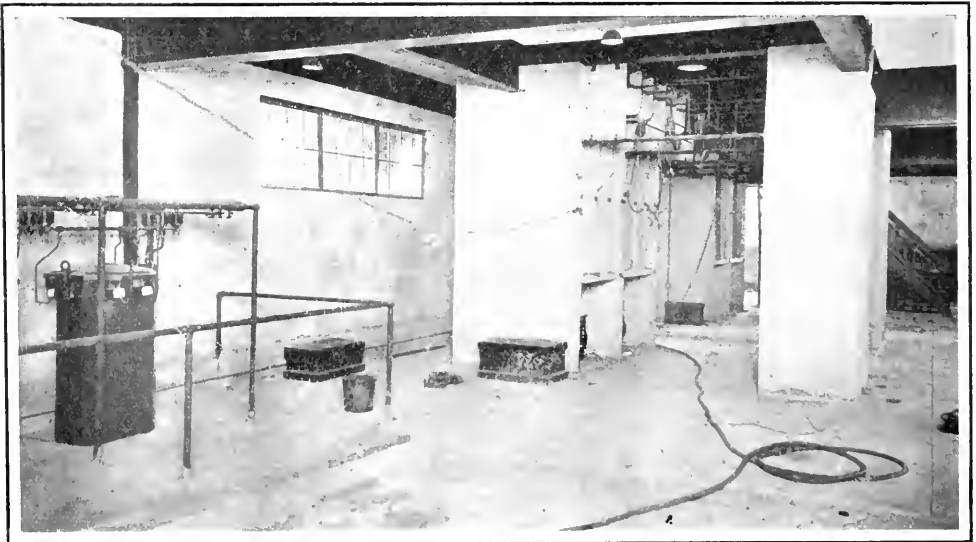
RANNEY FALLS DEVELOPMENT - CENTRAL ONTARIO AND TRENT SYSTEM Generating station equipment: Low-voltage (6,600 volts) bus-structure. July 1, 1922
