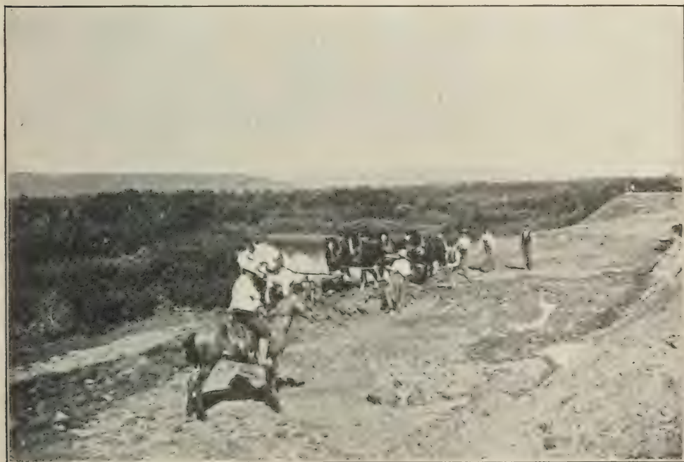
DOUKHOBORS AT WORK GRADING MAIN LINE. GRAND TRUNK PACIFIC RAILWAY.
