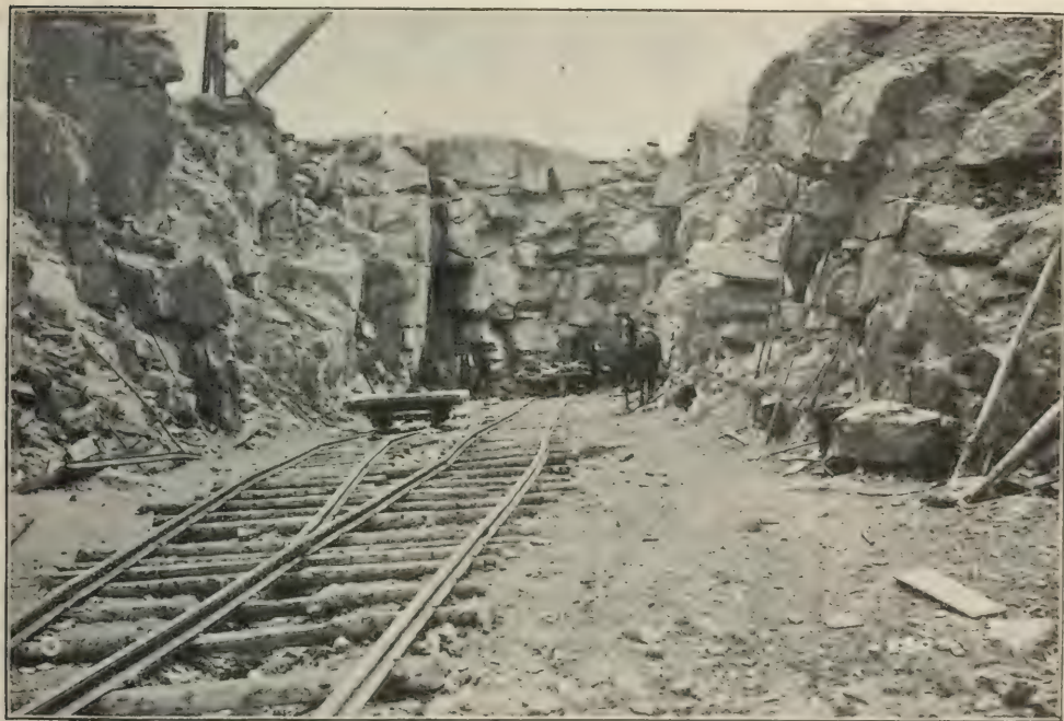
ROCK CUT ON THE MAIN LINE. GRAND TRUNK PACIFIC RAILWAY.
