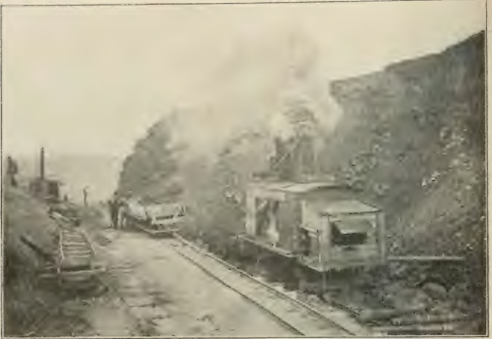
STEAM SHOVEL AT WORK, MAIN LINE, GRAND TRUNK PACIFIC RAILWAY.
