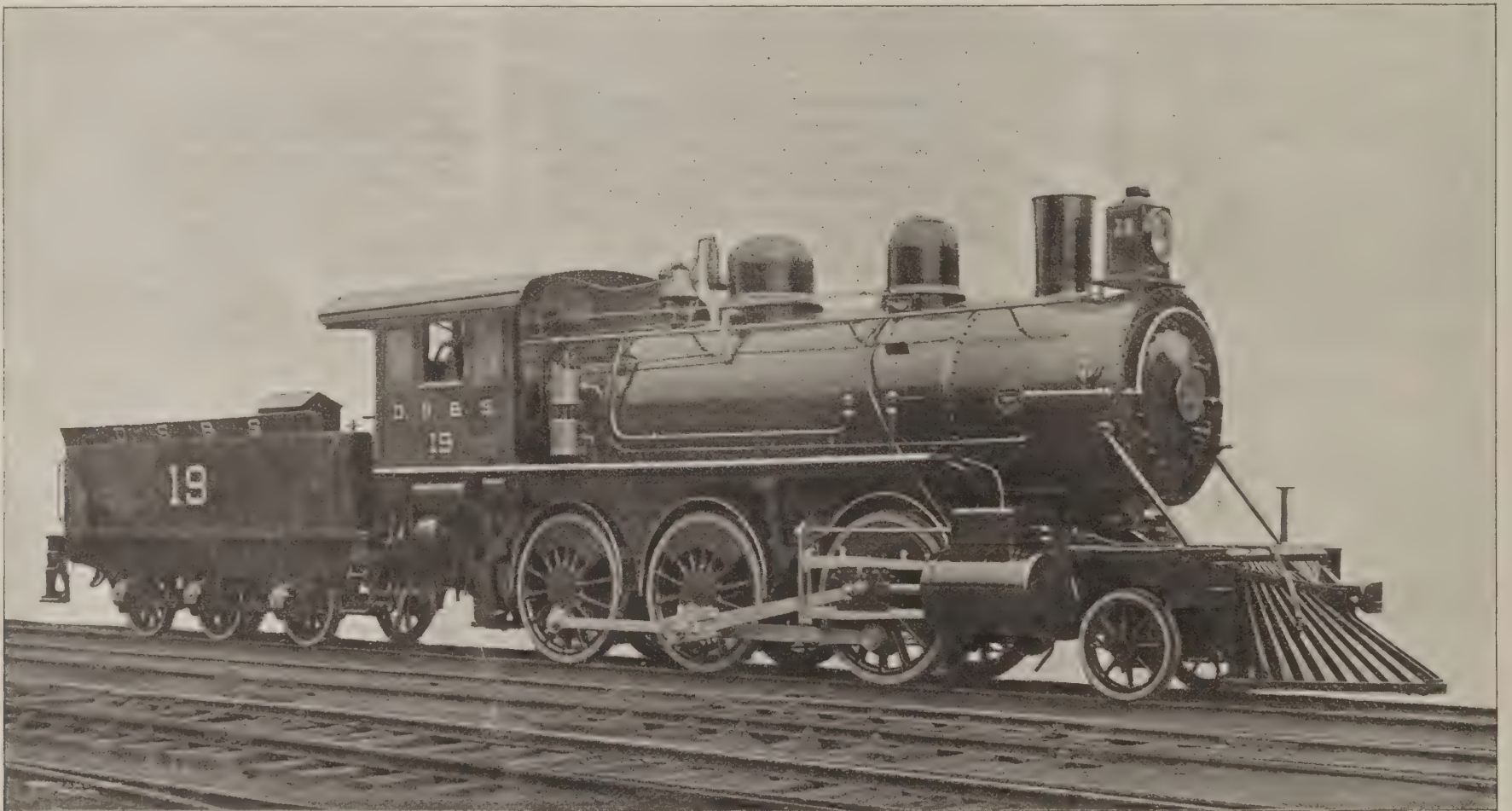
LARGEST MOGUL LOCOMOTIVE IN THE WORLD—DELAWARE SUSQUEHANNA & SCHUYLKILL RAILROAD.
