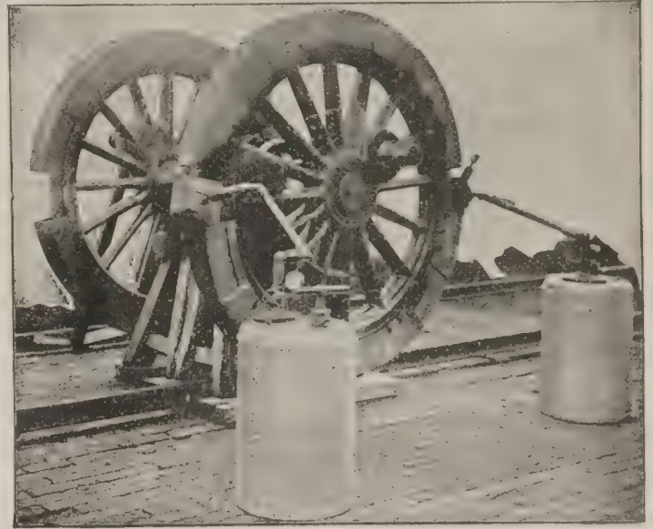
Fig. 98.—Wells Light Arranged to Heat Tires.
