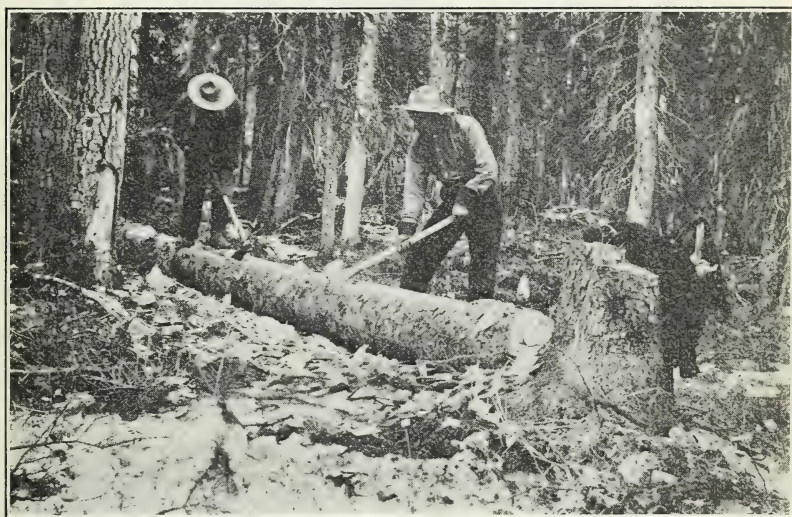
FIG. 21.—Hewing a water trough out of a spruce tree for improvement of soft-water spring, Montezuma National Forest
