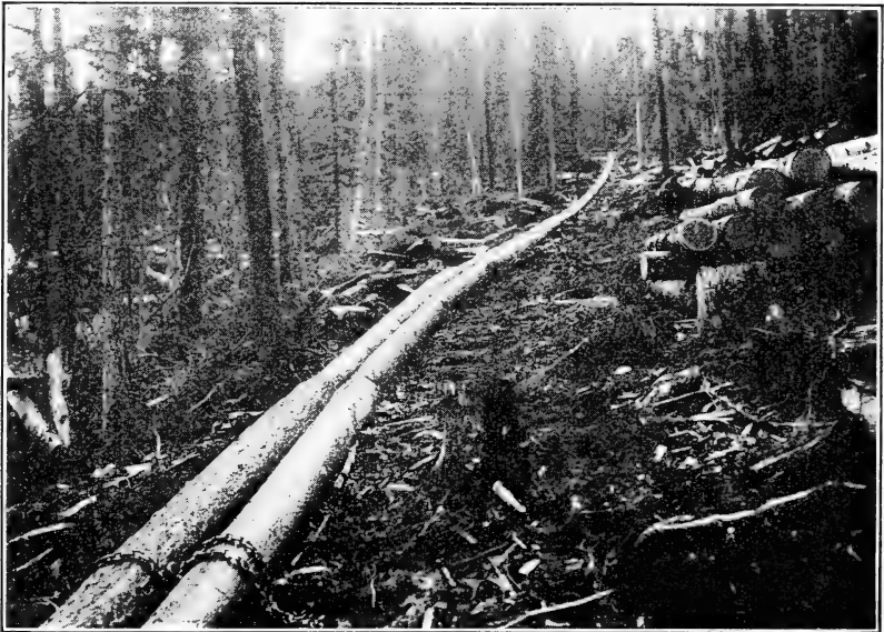
FIG. 11.—A skidway and log chute in the Arapaho National Forest
