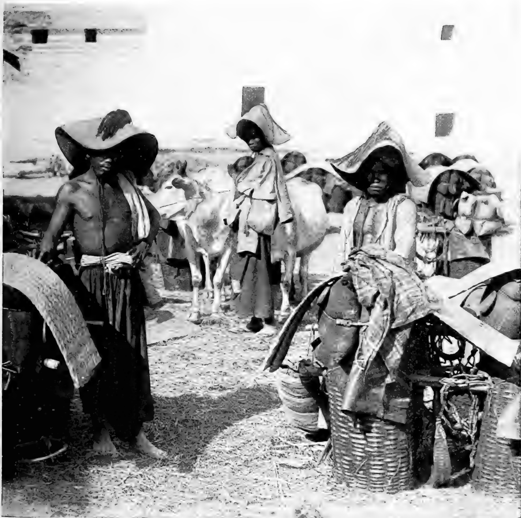
SHANS LOADING COMMISSARIAT STORE
