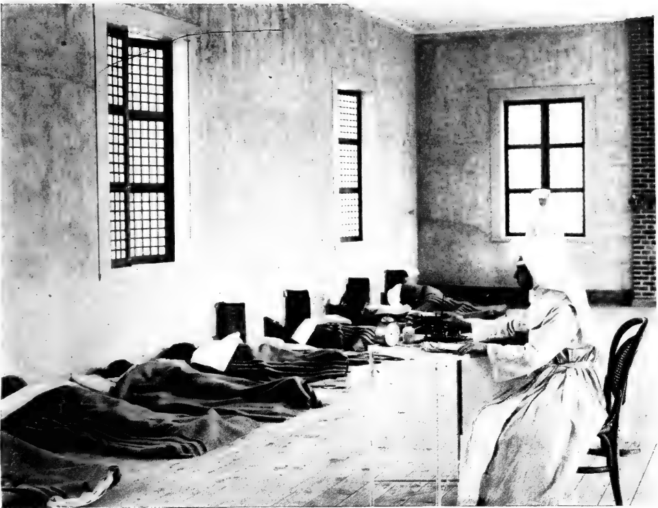
IN THE NEW HOSPITAL AT BONTOC
