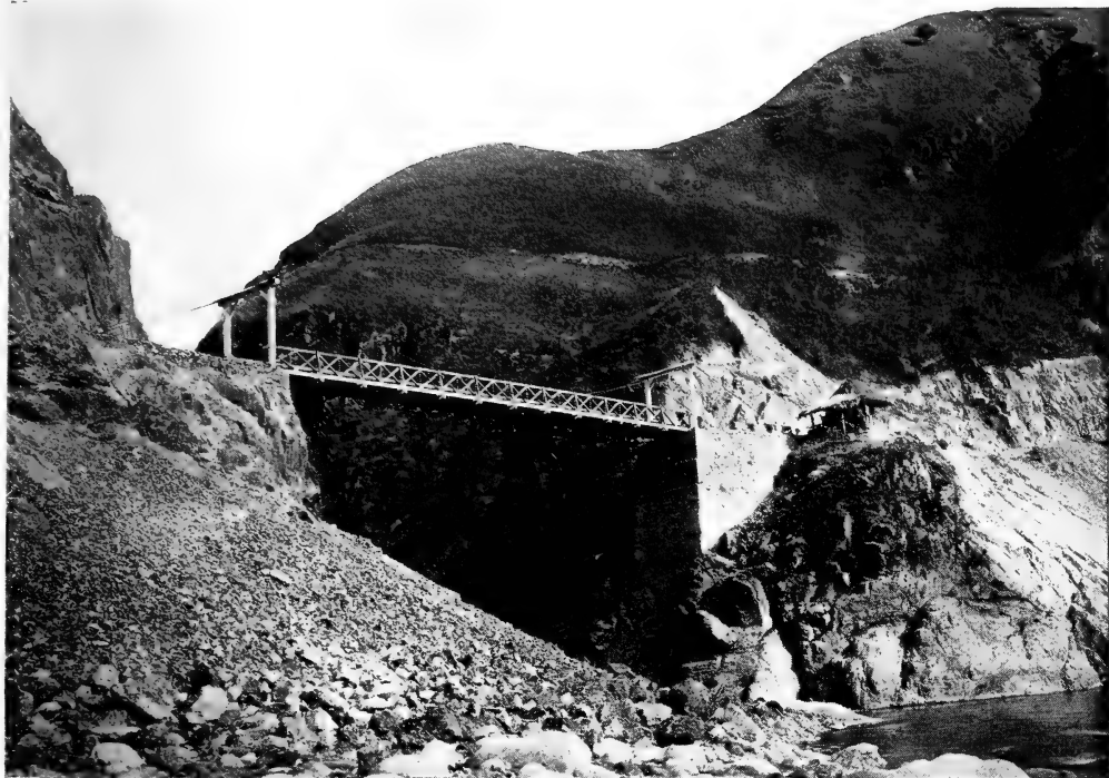
A MOUNTAIN PROVINCE BRIDGE BUILT UNDER AMERICAN RULE
