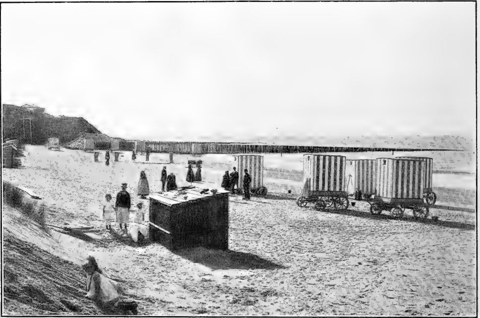
Pile Dikes for Protection against Marine Erosion
