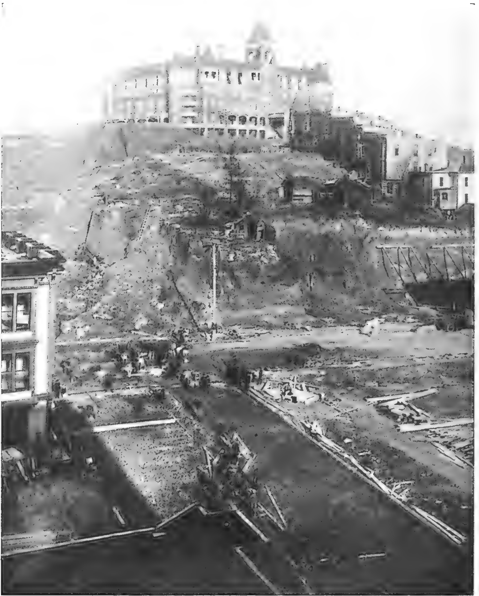
This and the succeeding three pictures show what is being done in Seattle in the way of removing hills for the expanding business district. These regrading projects involve the removal of more dirt than any other modern enterprise outside of the Panama Canal. The total depth of the excavation, from the foundation of the Old Washington Hotel, shown in this view, to the foundation of the New Washington, was 108 feet.
