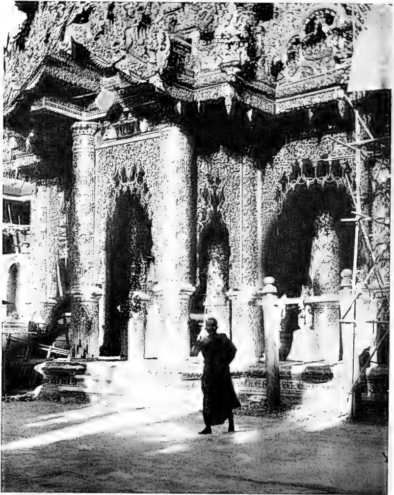
DETAIL OF CARVING ON AN ENTRANCE TO A CHAPEL
