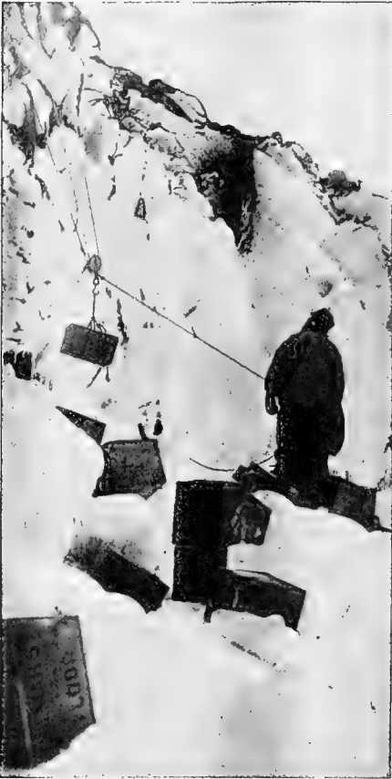
DERRICK POINT, SHOWING THE METHOD OF HAULING STORES UP THE CLIFF
