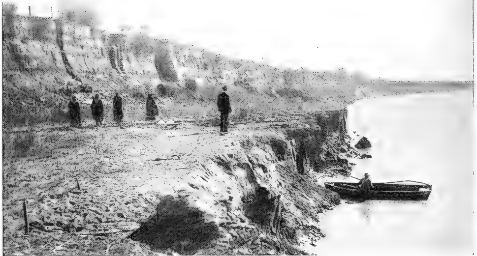
END OF THE PROTECTIVE LEVEE AT THE INTAKE OF THE IMPERIAL CANAL SYSTEM BELOW YUMA. CUT THROUGH AND DESTROYED BY THE COLO- RADO RIVER IN DECEMBER, 1906
