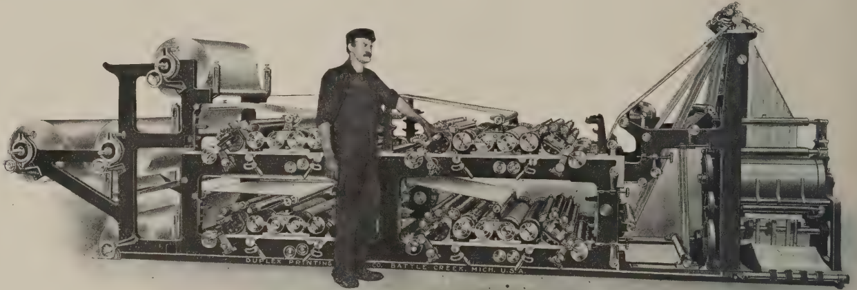
DUPLEX TUBULAR SINGLE-PLATE 16-PAGE PRESS
