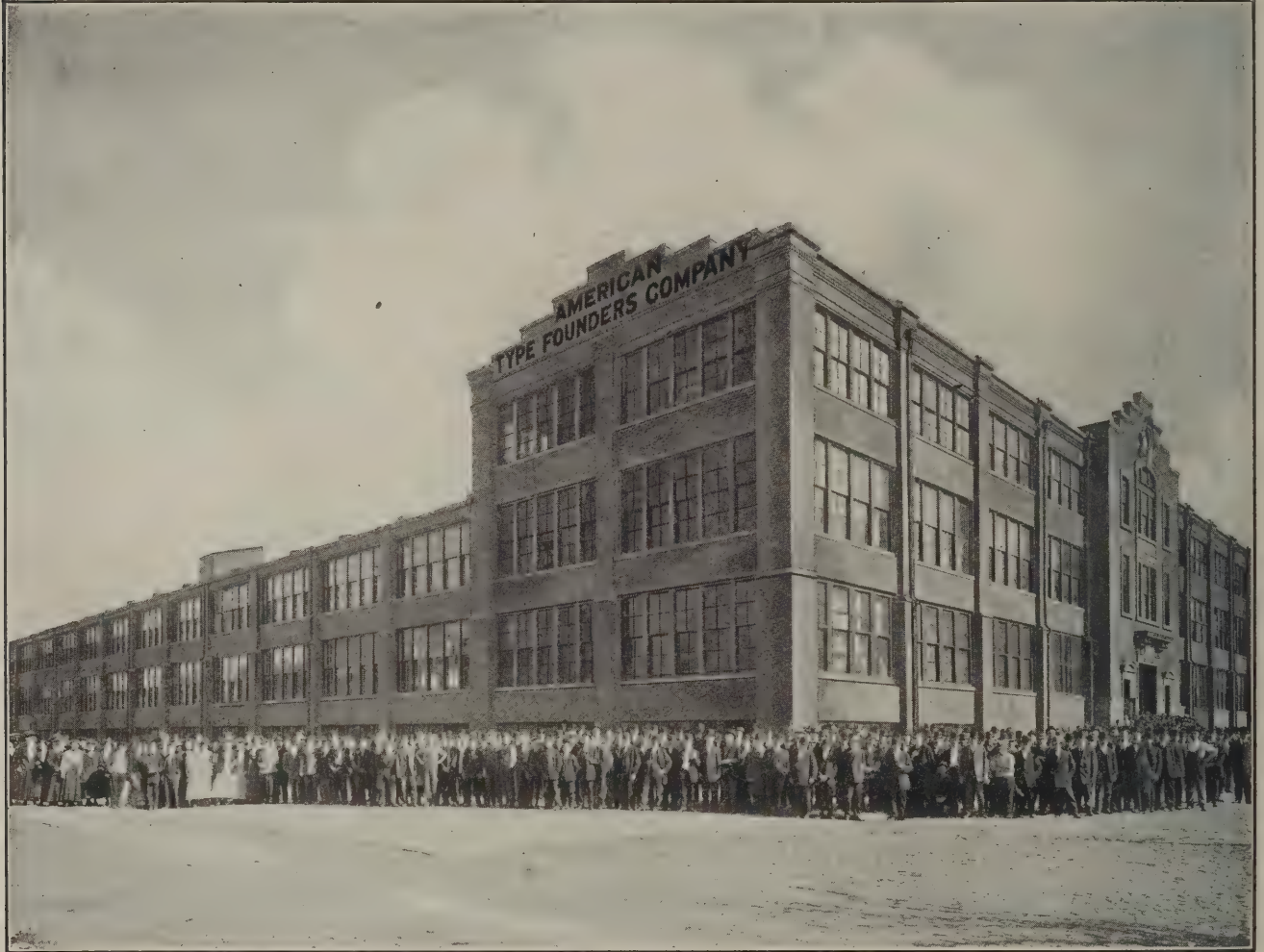
CENTRAL PLANT AMERICAN TYPE FOUNDERS COMPANY
