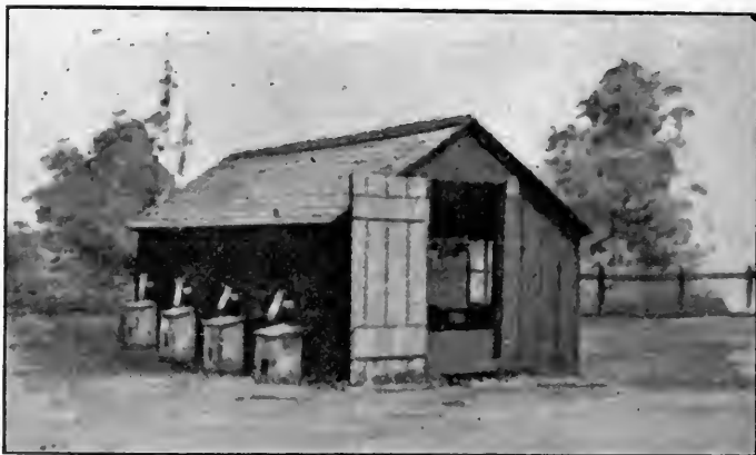
Combination colony brooder-house, breeding or laying pen. The house in illustration is 8 feet deep and 16 feet long, and will accommodate up to 300 chicks; is built upon two 4 x 4-inch runners, and has two sliding windows in front. Can be used as a primary brooder till chicks are past the danger-point, i.e., the first fourteen days; and they can then be removed to colony houses on free range. When used for this purpose, the house can be stationed close to farm buildings and enable rancher to pay more attention to chicks with less labour and time than when they are out on free range.
