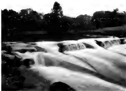
Water from Bussell Branch contributes to the output of Arkansas’s Mammoth Spring, whose waters cascade over a dam built in 1888 from hand-quarried limestone.
